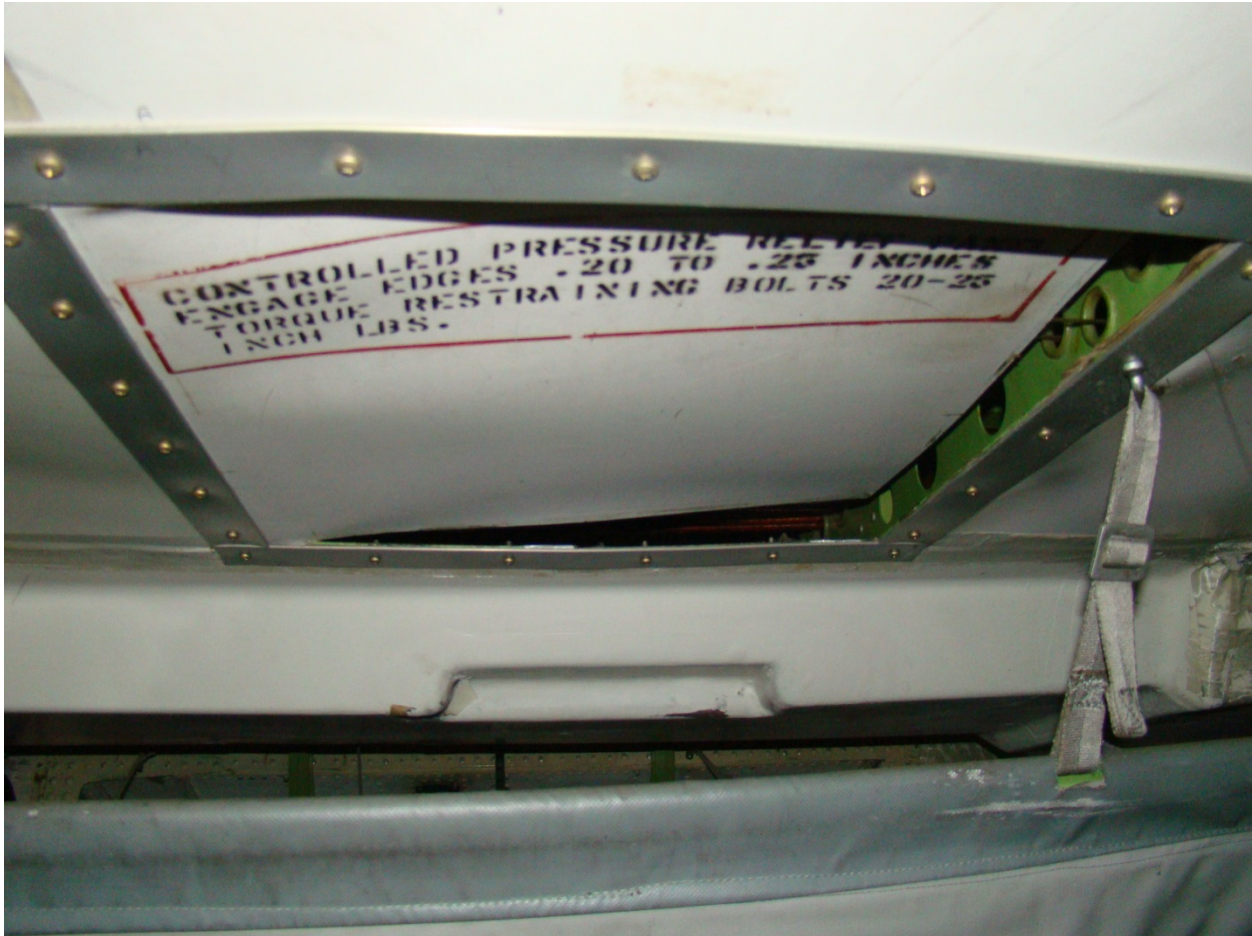
Figure 12. Pressure relief panel above the door after a 6.4 cell at 100% and a 20 cell at 50%
