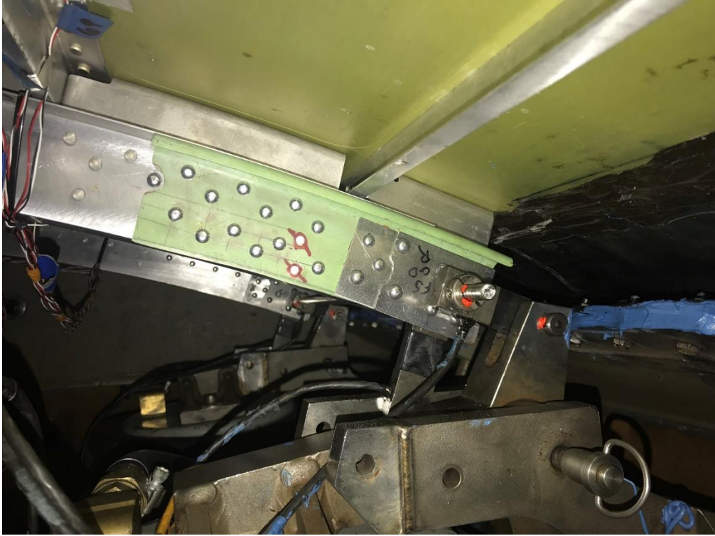
Figure 60. Picture of frame end repair at frame
