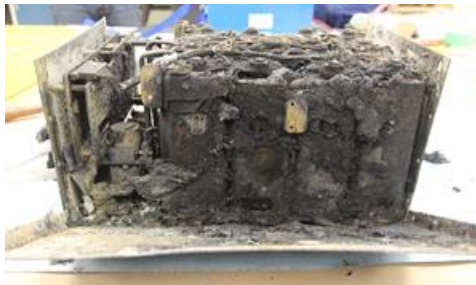
Figure 1. An example of a catastrophic failure of a large lithium-ion battery, initiated by a thermal runaway of a single cell and subsequent chain reaction of failure propagation
