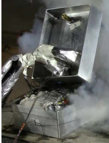
Figure 40. Overcharged edge cell pair caused the battery box lid to be blown off, resulting in cell effluence rapidly venting to ambient
