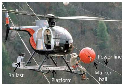
Figure 4.16: Installing Markers on Power lines 27
