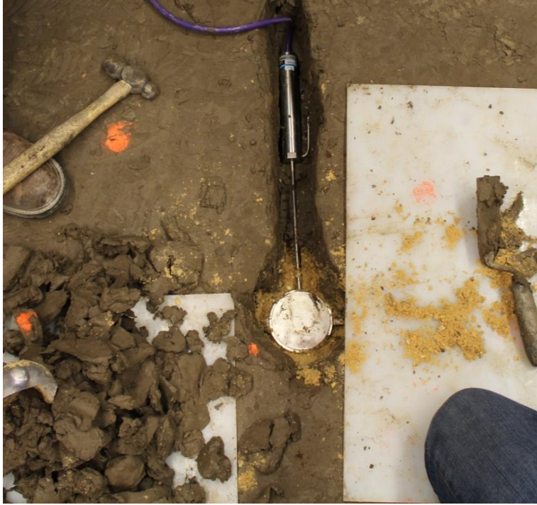
Figure 11. Subgrade EPC Installation
