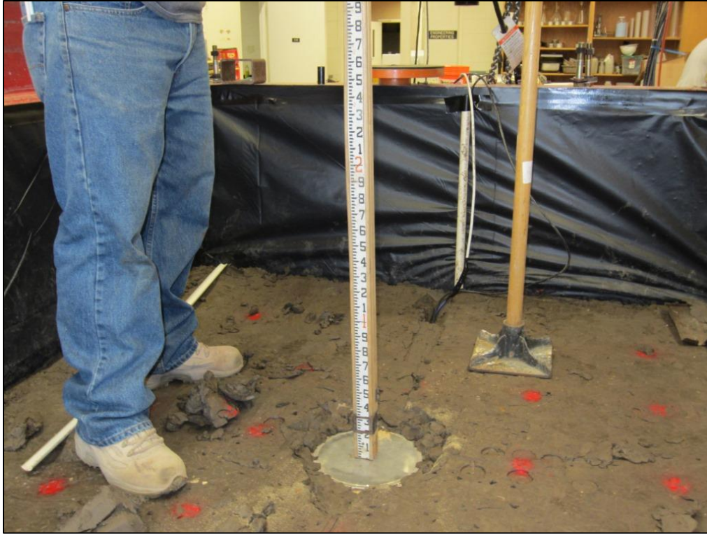
Figure 35. Determining Elevation of Installed EPC
