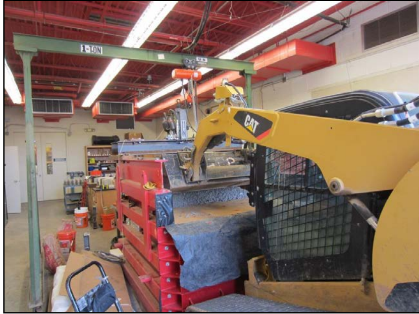
Figure 20. Placement of Base-Course Material
