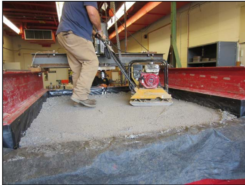
Figure 21. Compaction of the Aggregate Base Course Using Vibratory Plate Compactor
