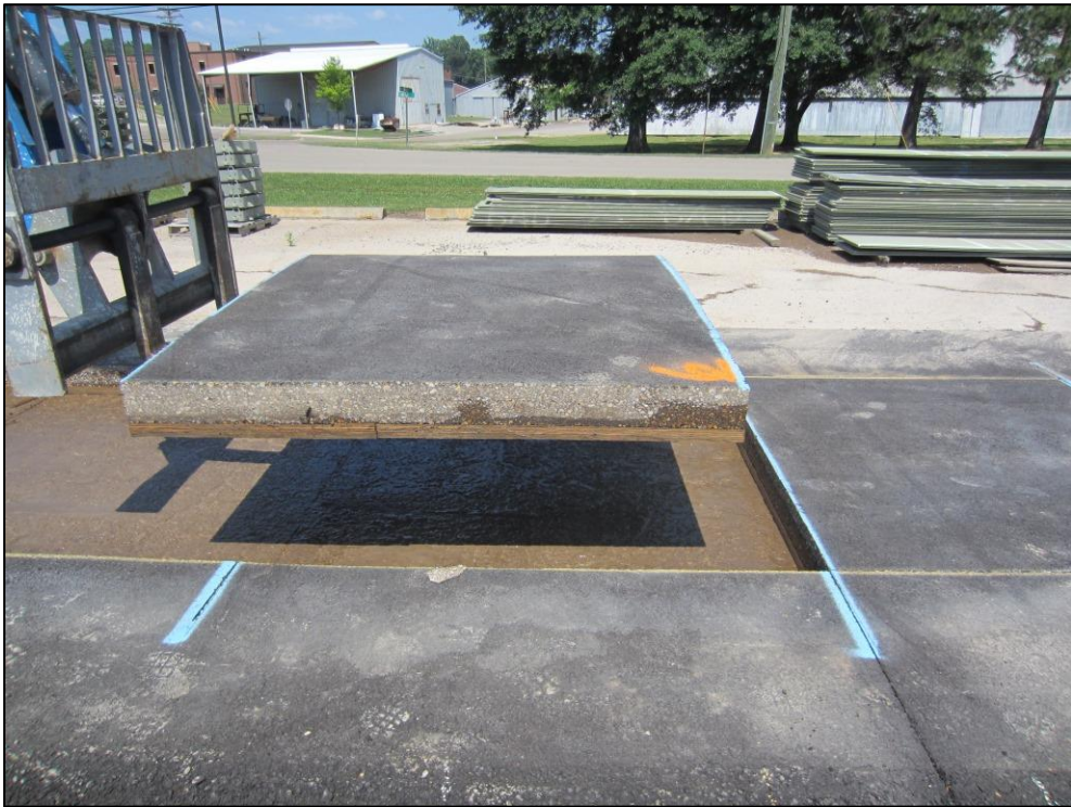
Figure 29. The HMA 5.5- by 5.5-ft Slab
