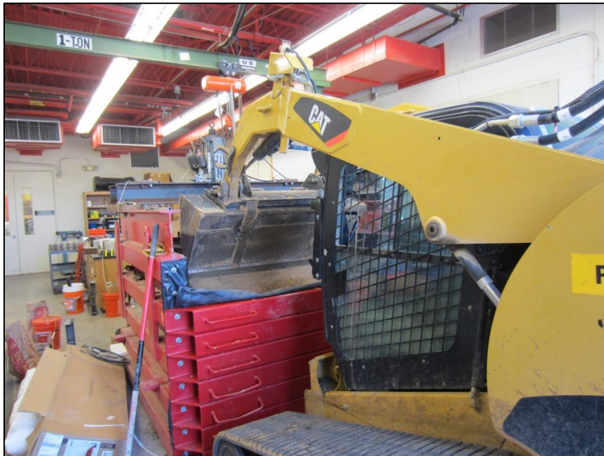
Figure 16. Subbase Material Placement
