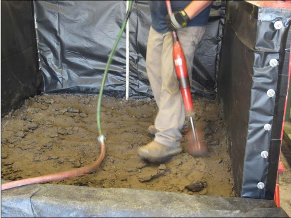
Figure 12. Compaction of Subgrade Material
