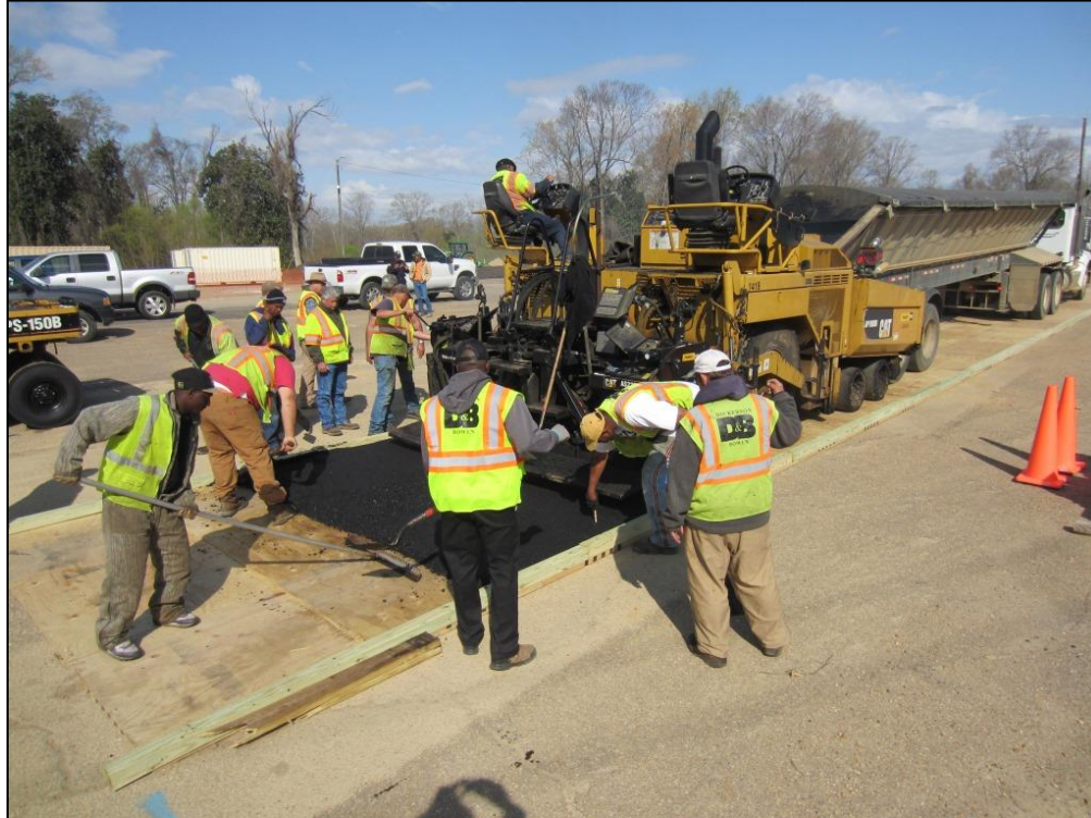
Figure 27. Initial HMA Placement
