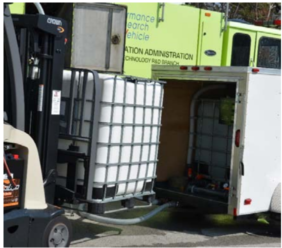
Figure 21. NoFoam Tank Level Test Connection
