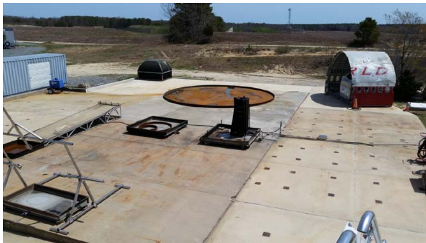
Figure 1. The FAA Outdoor Fire Test Facility
