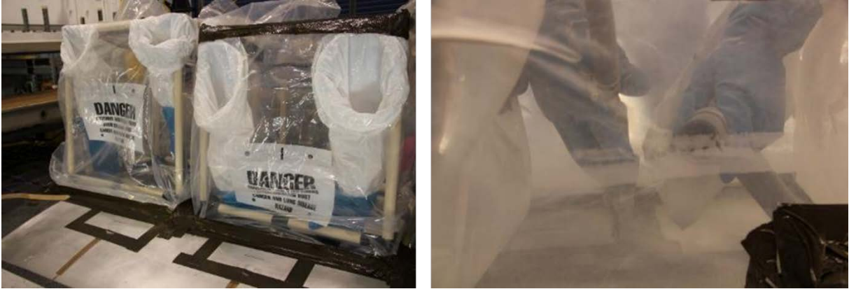
Figure B-2. Grit blasting
