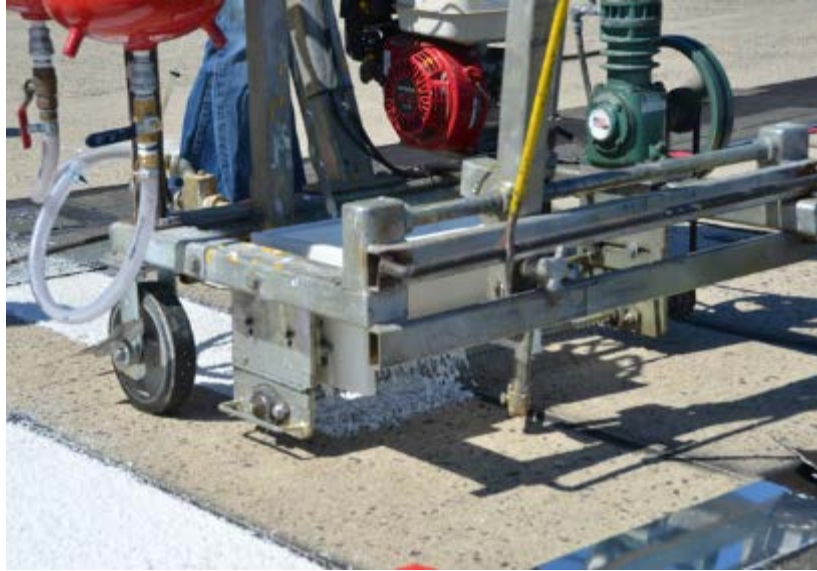
Figure 3. White SMMA Marking Installation at ACY
