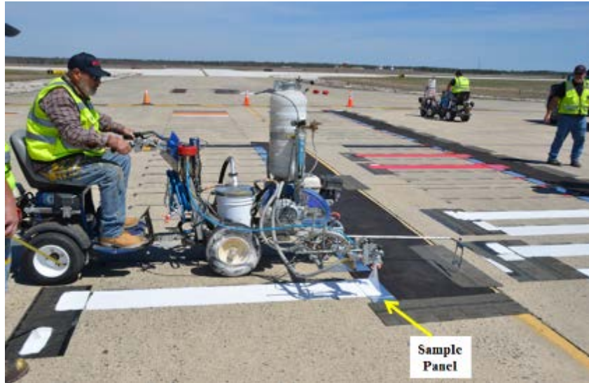
Figure 5. White Waterborne Type II Paint Application to Sample Panel
