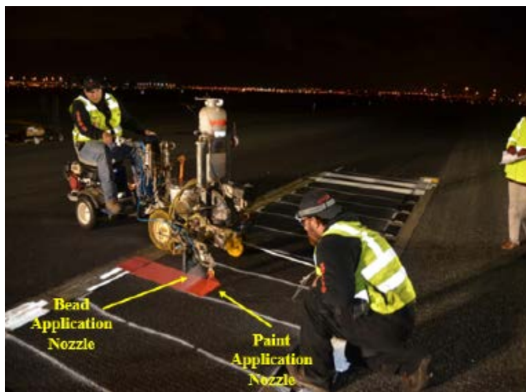
Figure 2. Red Waterborne Type I Marking Installation at EWR
