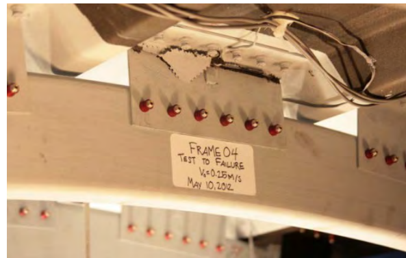
(b) Crushed Shear Tie
