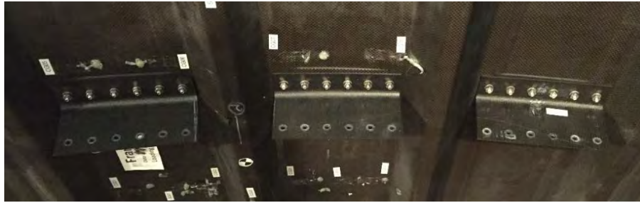
(b) C-frame only removed (shear ties mounted)
