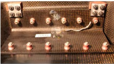
(c) Undamaged shear tie for baseline (ST11)
