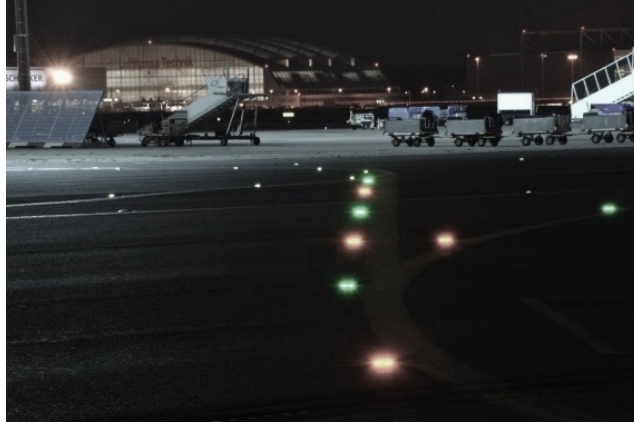
Figure 4. Color-coded taxiway centerline lights installed to enhance pilot situational awareness (source: Airfield and runway lighting, 2017)
