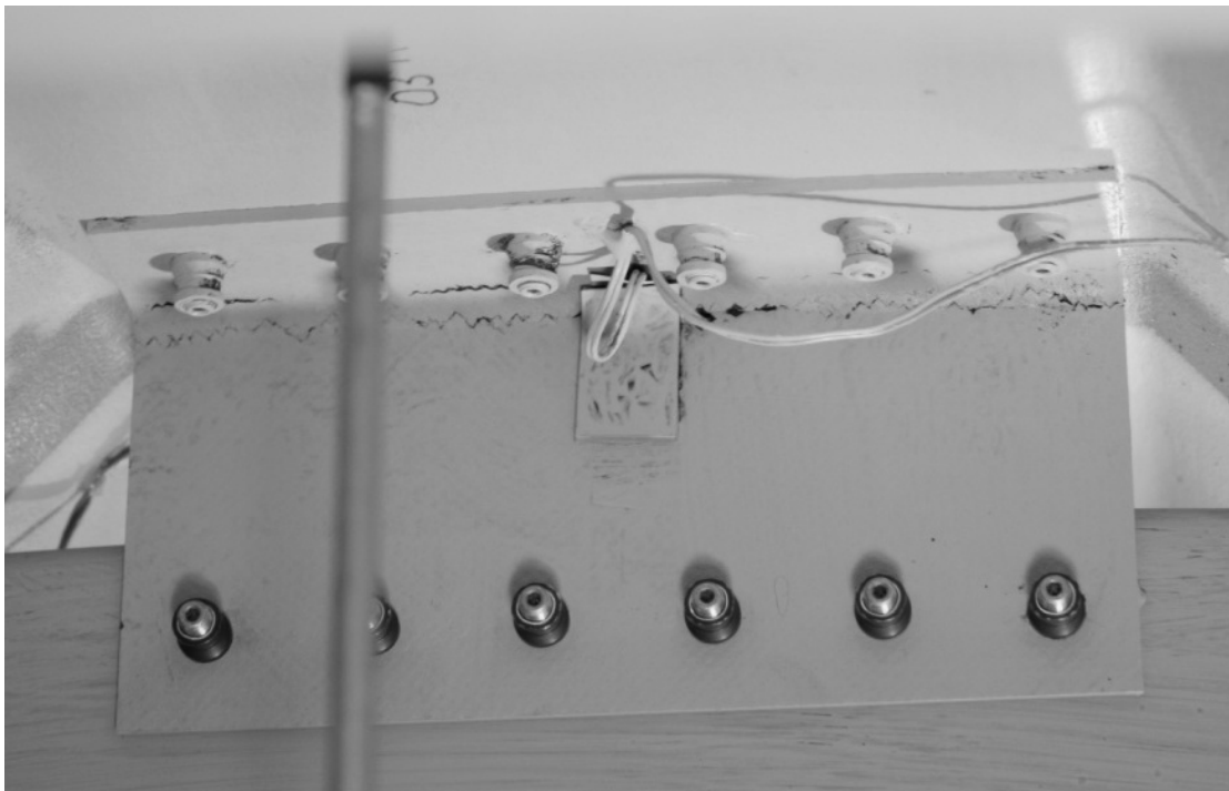
Figure 46. Shear-tie corner crushing failure after first loading of panel Frame03; shear tie painted white to visually accentuate cracks
