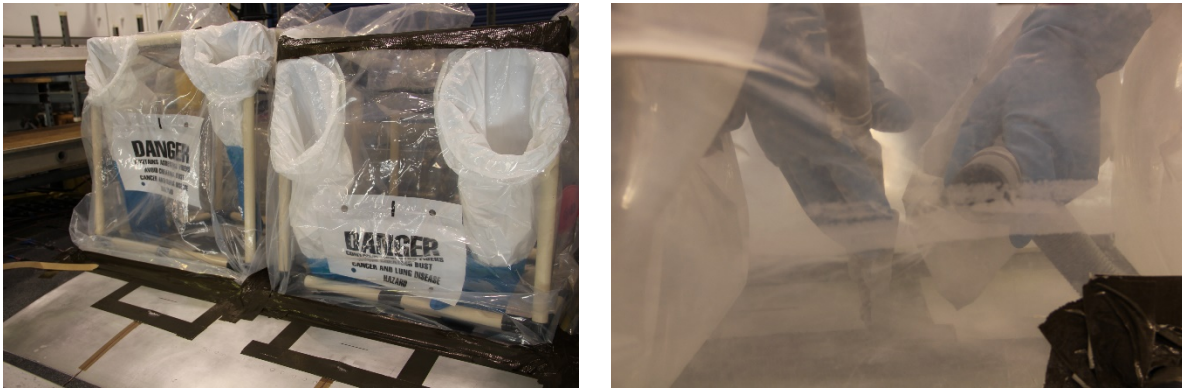
Figure D-1. Grit blasting
