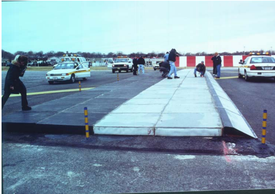
Figure 39. Visual Inspection of JBR Demonstration Blocks
