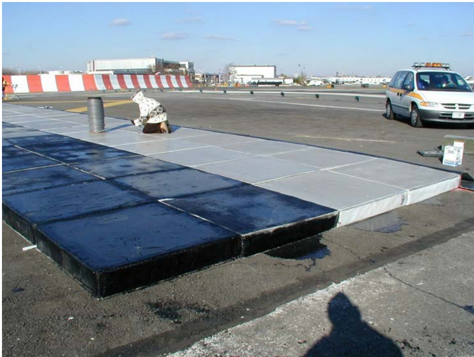
Figure 38. Polyurethane Coating at Front and Asphalt Coating at Rear
