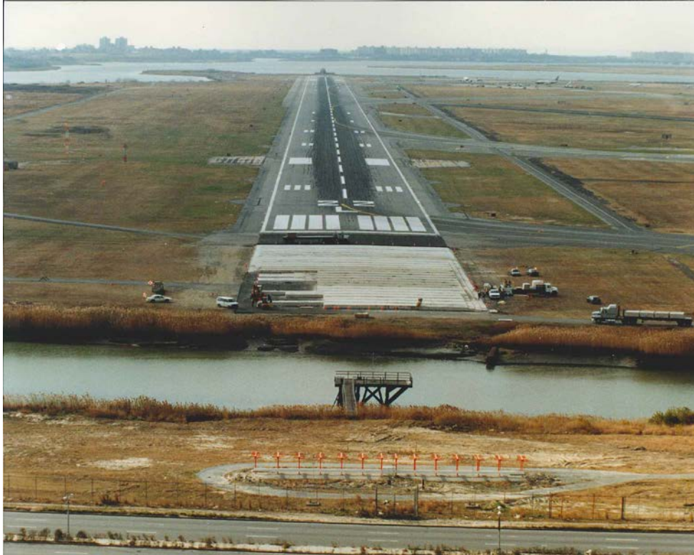
Figure 21. The EMAS Prototype Serving JFK Runway 4R
