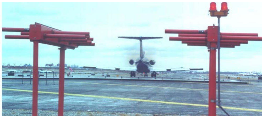
Figure 40. Dark Horizontal Strip is the Rear Face of the JBR Demonstration Bed (Runway 22 localizer is in the foreground.)
