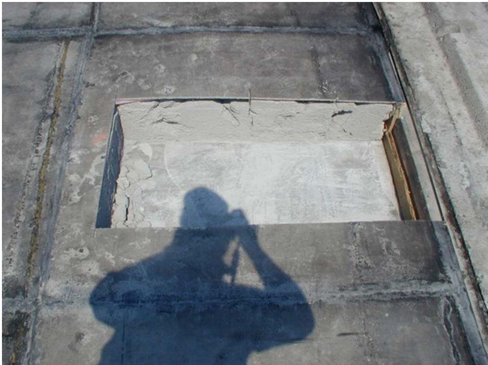
Figure 43. Full-Depth Section Removal From JBR System
