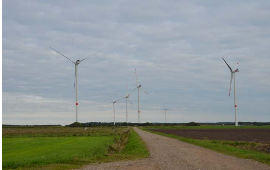
Figure 6. Wind Turbines at the Braderup Wind Park
