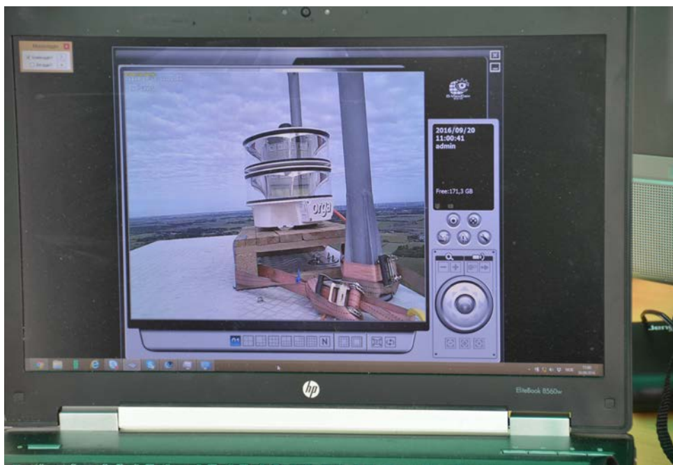
Figure 11. Camera Feed Used to Monitor Obstruction Light Status During Assessment
