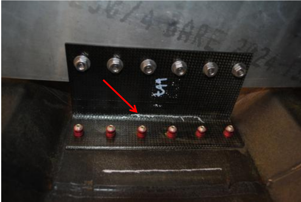
Figure 108. Crack on shear tie bend radius not detectable using NDI from front side of panel
