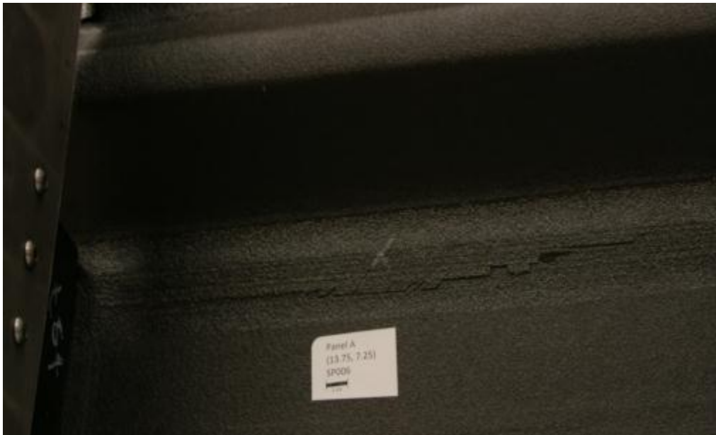
Figure 107. Stringer flange delamination detectable from backside of panel A
