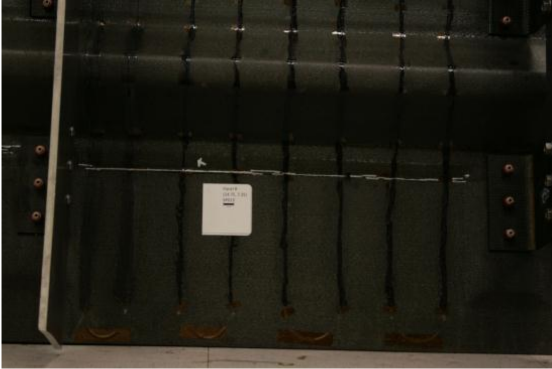
Figure 101. Broken FO due to stringer flange delamination
