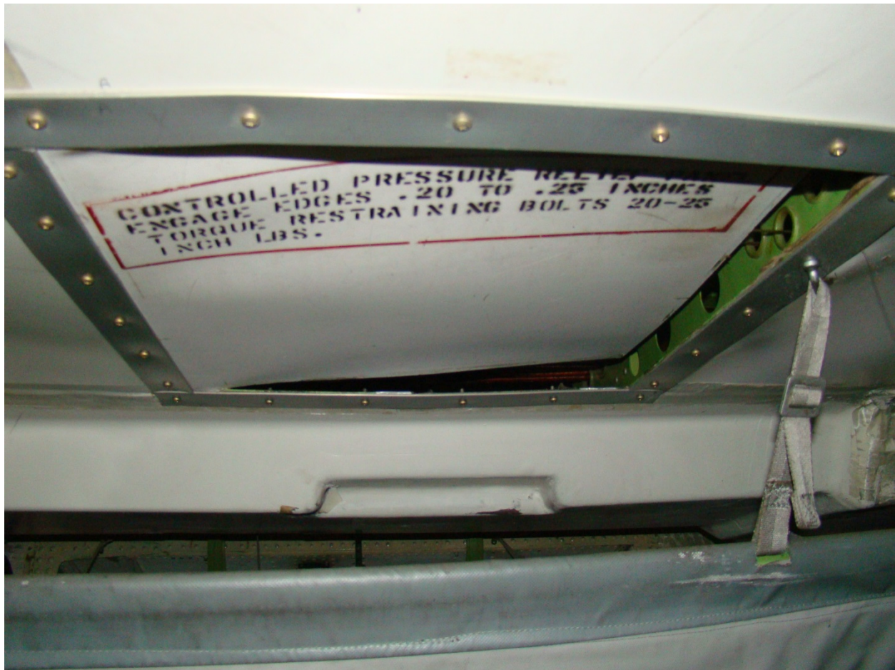
Figure 42. Pressure-relief panel above door after 6.4 cells at 100% and 20 cells at 50%
