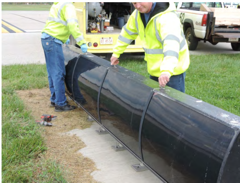
Figure 37. Installation of Proposed Sign Panels at CLE
