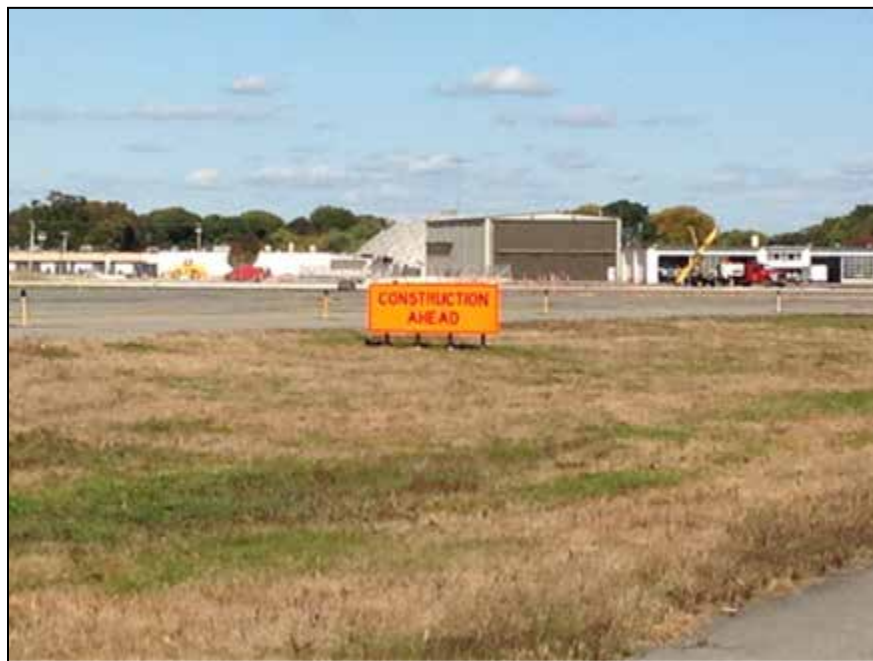
Figure 47. CONSTRUCTION AHEAD Sign on TWY T at PVD
