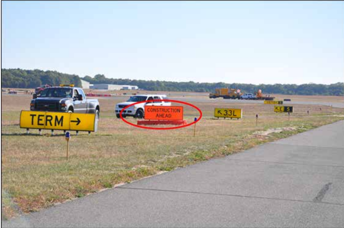
Figure 44. CONSTRUCTION AHEAD Sign From TWY S View at ISP
