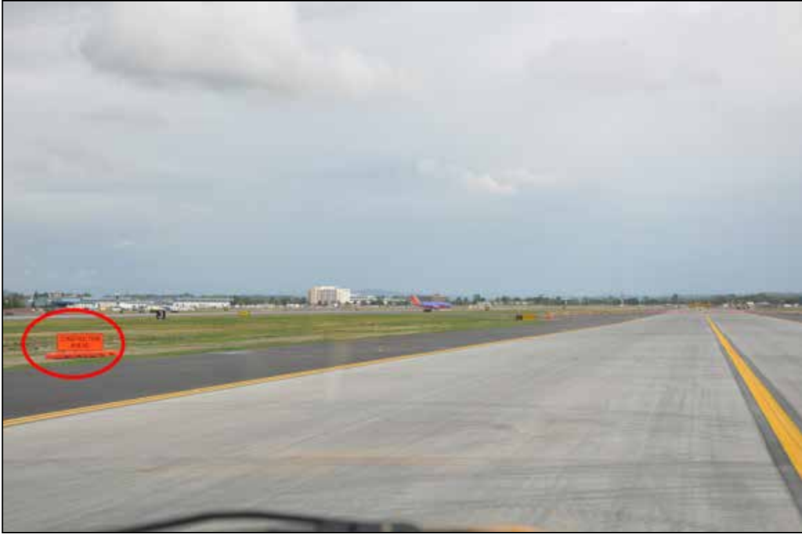
Figure 53. CONSTRUCTION AHEAD Sign on TWY C at PDX
