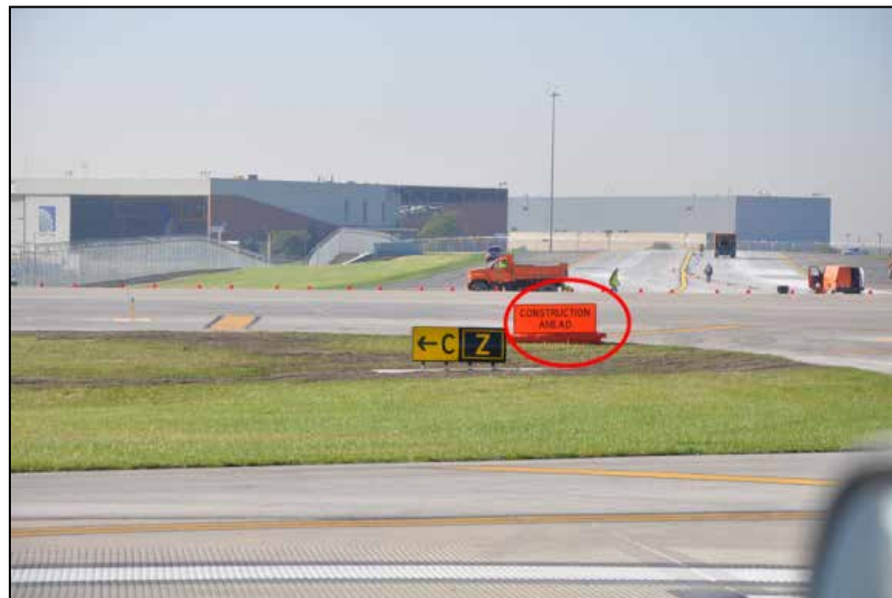
Figure 51. CONSTRUCTION AHEAD Sign on TWY Z at ORD
