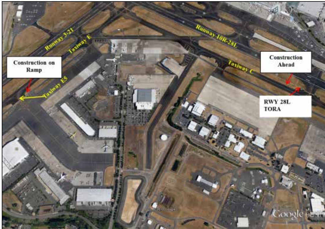
Figure 52. Overview of Safety Orange Construction Sign Locations at PDX
