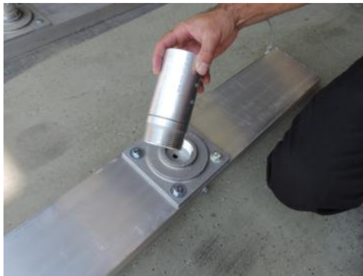
Figure 38. Base Stand and Frangible Coupling
