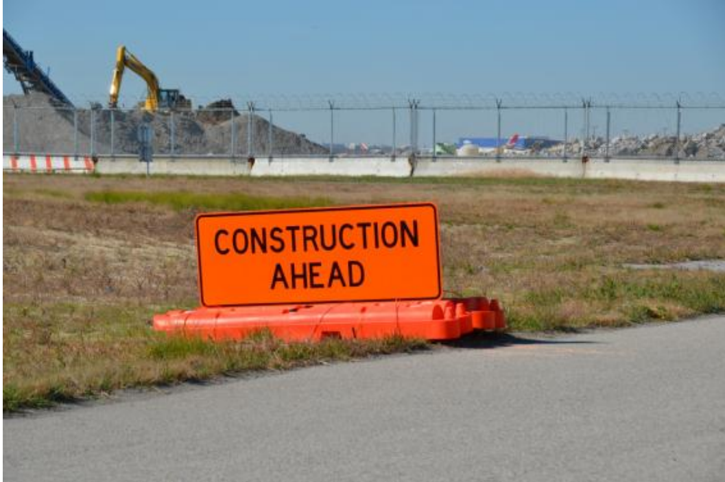
Figure 61. CONSTRUCTION AHEAD Sign at JFK
