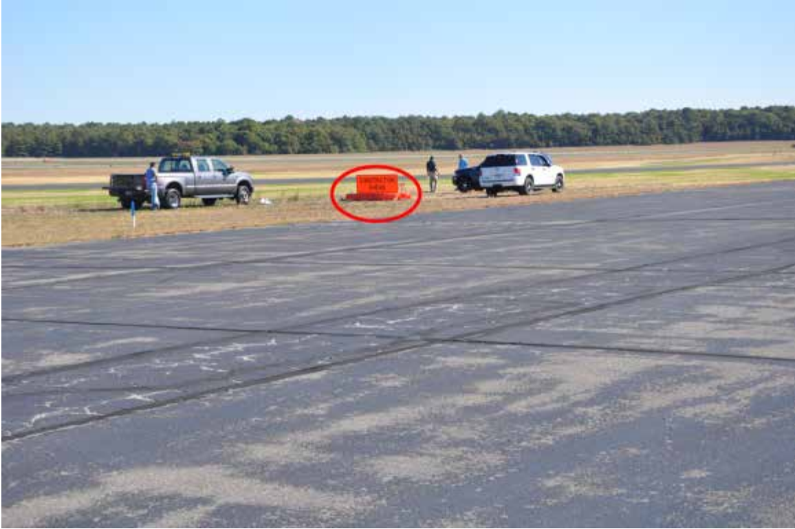
Figure 45. CONSTRUCTION AHEAD Sign as Observed on RWY 10 at ISP
