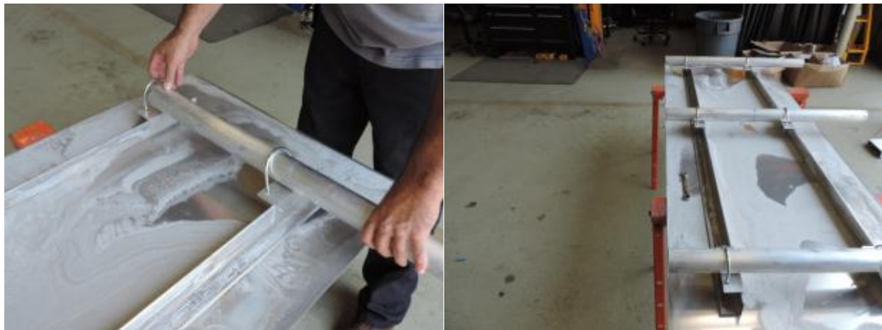
Figure 40. Attachment of Legs to Sign Panel
