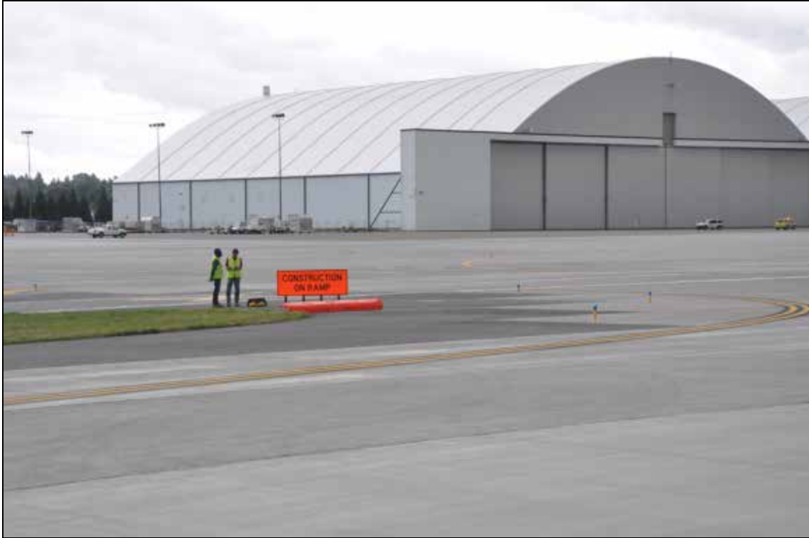
Figure 55. CONSTRUCTION ON RAMP Sign at PDX
