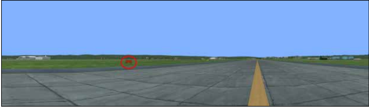
Figure 23. Run 4 Simulated CONSTRUCTION 600 FT AHEAD Sign During Daytime Conditions
