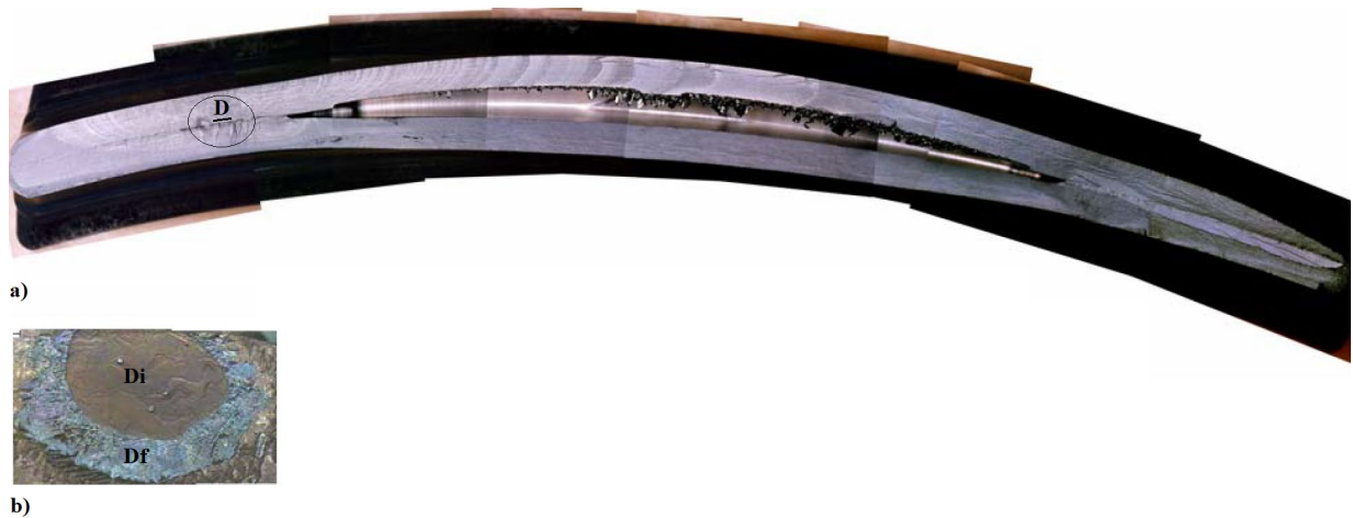
Figure 7. Failed blade: a) Cross-section showing the disbond (D); b) Initial (Di) and final disbond (Df) shape [124] (modified).
