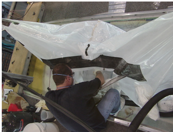
Figure D-1. Grit-blasting the patch region
