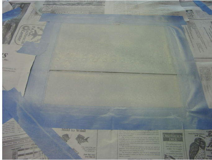
Figure D-4. Patch region just after application of bond-primer
