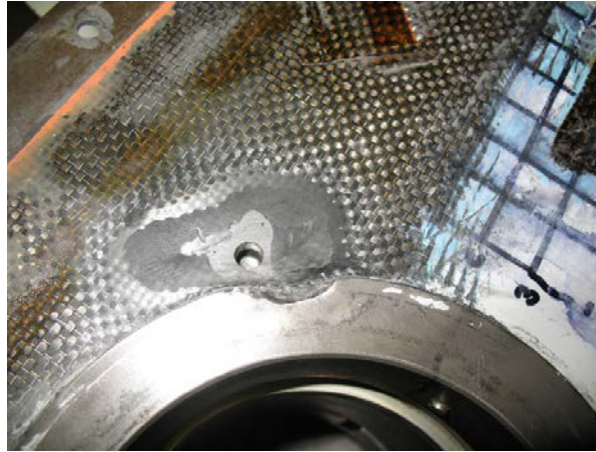
Figure 87. Hole repair after 1.5-DLT inspections
