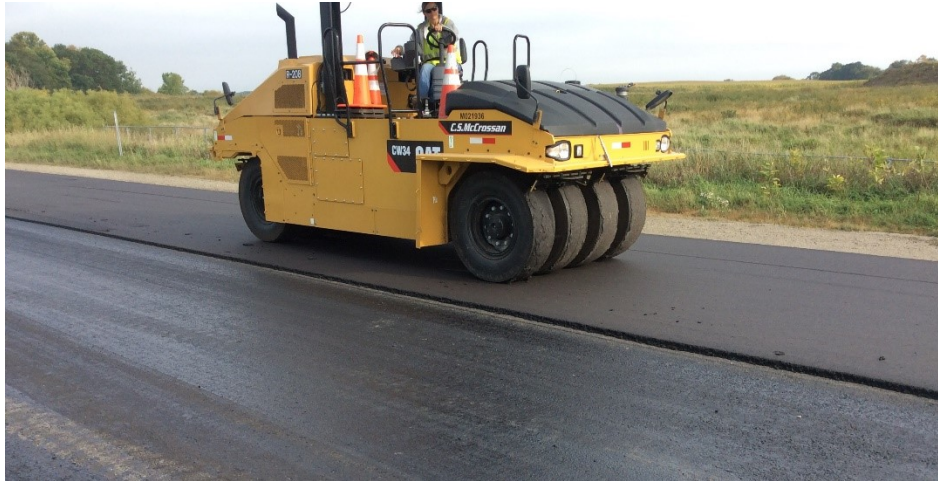
Figure 7 Compacting the paved HMA surface on MnROAD Cell 135
