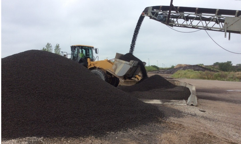
Figure 3 Contractor processing RAP used in the MnROAD CCPR test sections
