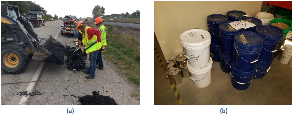
Figure 9 (a) MnDOT engineers reserving CCPR field mix materials at MnROAD and (b) reserved MnROAD CCPR materials in the laboratory for test specimen preparation
