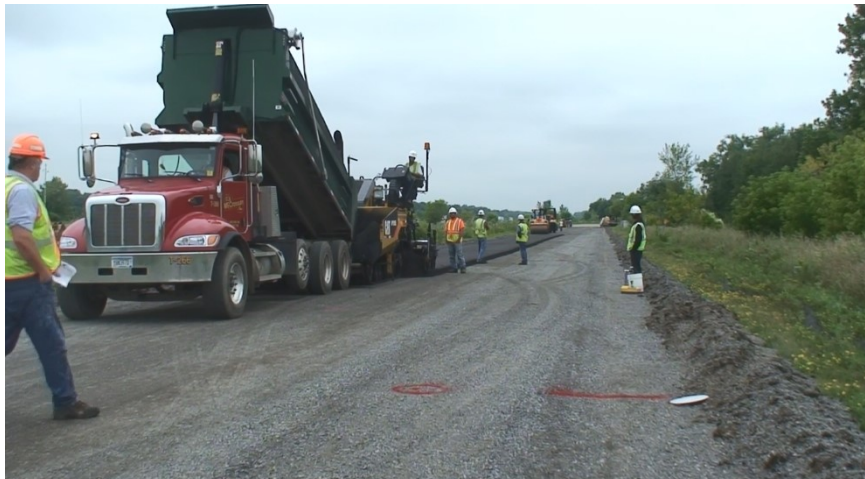
Figure 4 Laydown of CCPR mixture for MnROAD Cells 133, 233, 135, and 235
