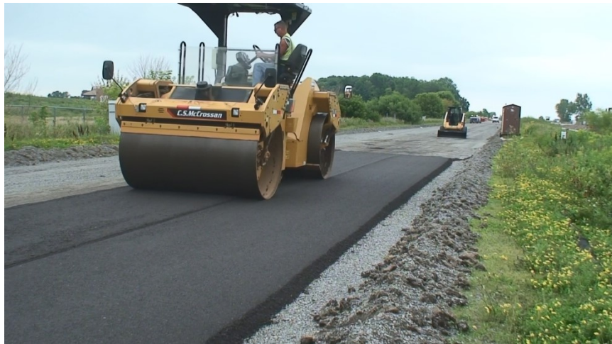
Figure 6 Compaction of placed CCPR on MnROAD Cells 133, 233, 135, and 235
