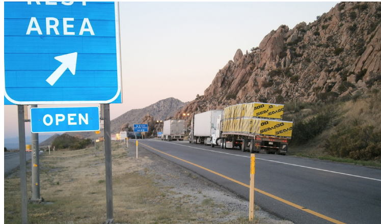
Figure 1: Truck Parking on Ramp, Texas Canyon Rest Area, AZ
