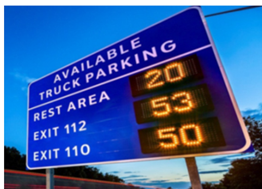
Figure 9: Example Dynamic Parking Capacity Sign
