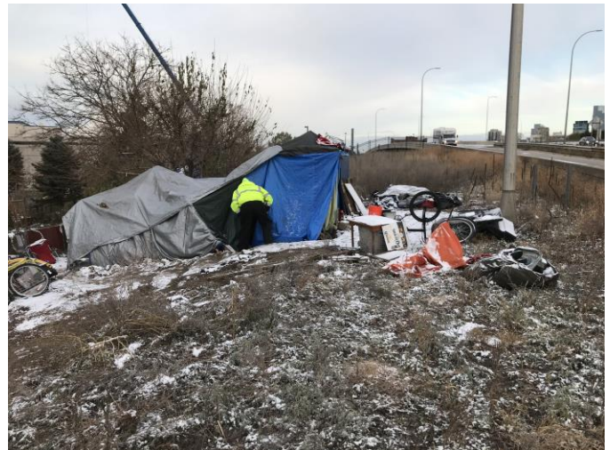
Figure 1. Maintenance work within homeless camp within the ROW
