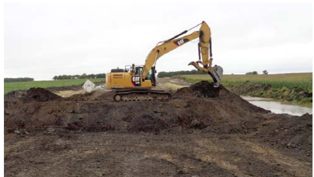
Backfilling transition zone (blending new with insitu material)
