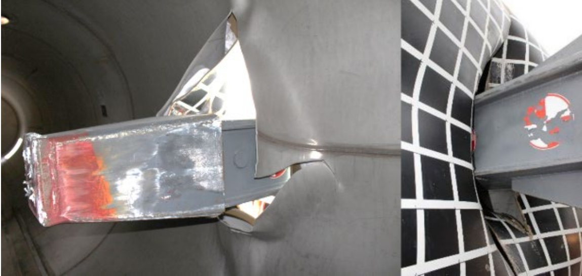
Figure 21. Interior (left) and Exterior (right) Views of Tank Damages from East Side (Prior to Impactor Removal)
