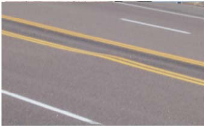
Figure 2 – Pavement Heaves
