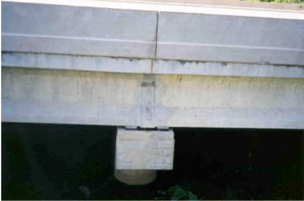
Figure 18. Watson Creek Bridge (East Bound): Un-cracked continuity joints (bridge No.1130-153).
