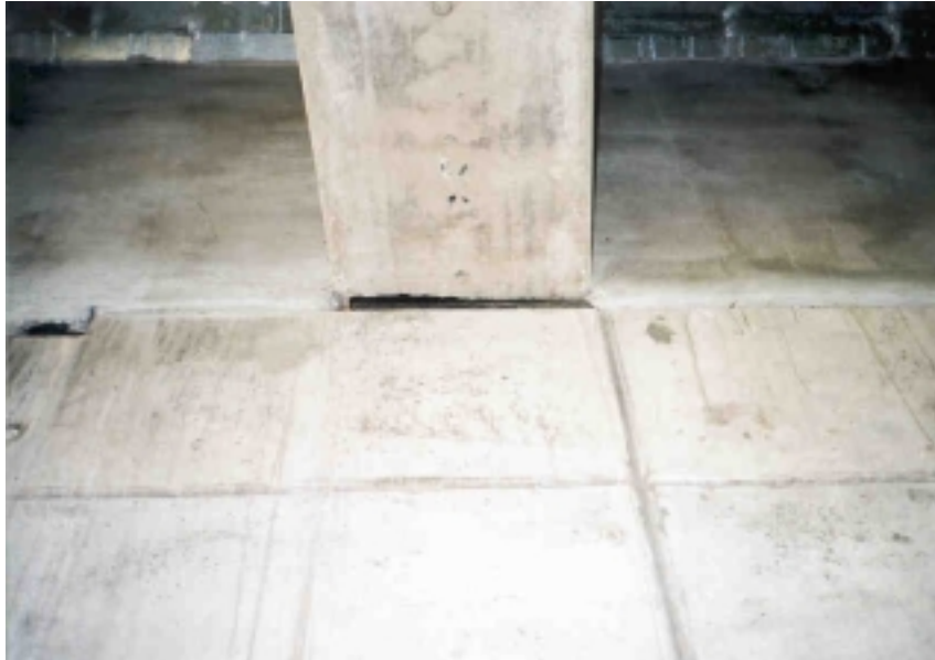
Figure 113. End diaphragm (Bridge No.1143-176).
