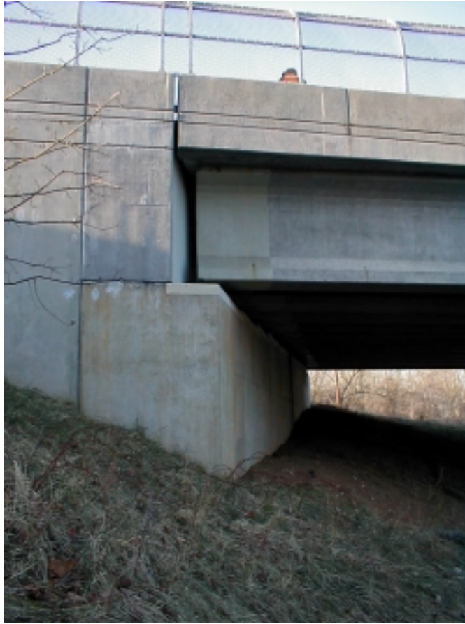
Figure 96. Girder end condition at the abutment (Bridge No. 1013-151).
