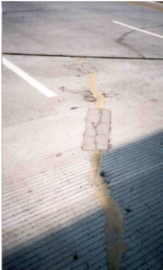
Figure 108. Repaired transverse crack (Bridge No. 1143-170).
