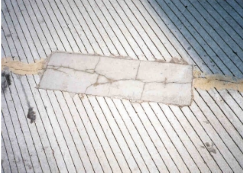
Figure 109. Close up view of repair patch (Bridge No. 1143-170).
