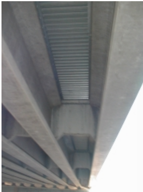
Figure 95. A view from underneath the bridge (Bridge No. 1013-151).
