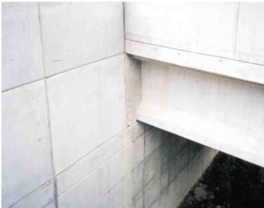
Figure 105. Girders embedded in end diaphragm (Bridge No.1143-168).
