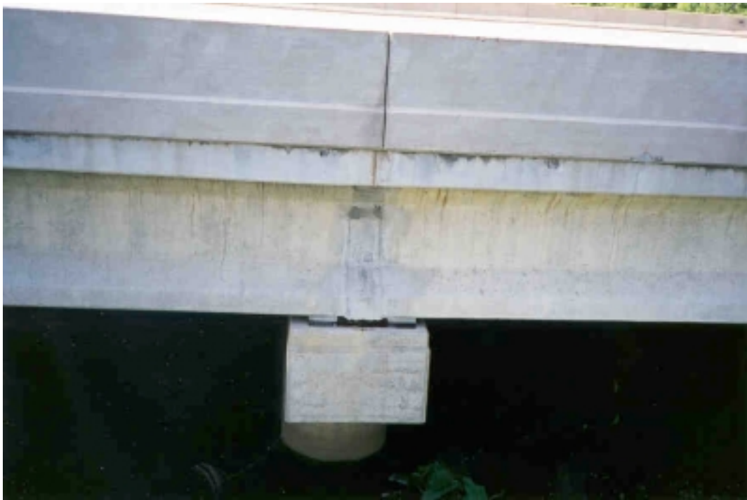
Figure 101. Un-cracked continuity joint (Bridge No.1130-153).
