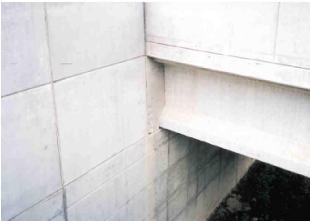
Figure 10. Boundary condition: girders are bounded.
