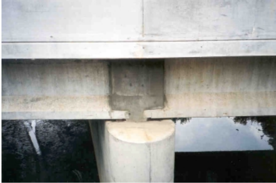
Figure 106. Continuity joint (Bridge No. 1143-168).
