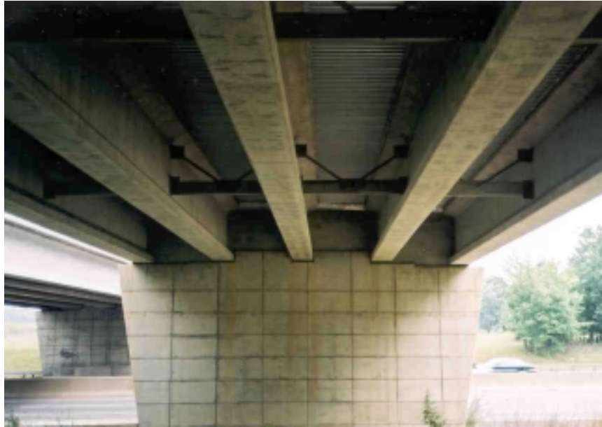
Figure 114. A view from underneath the bridge (Bridge No.1143-176).
