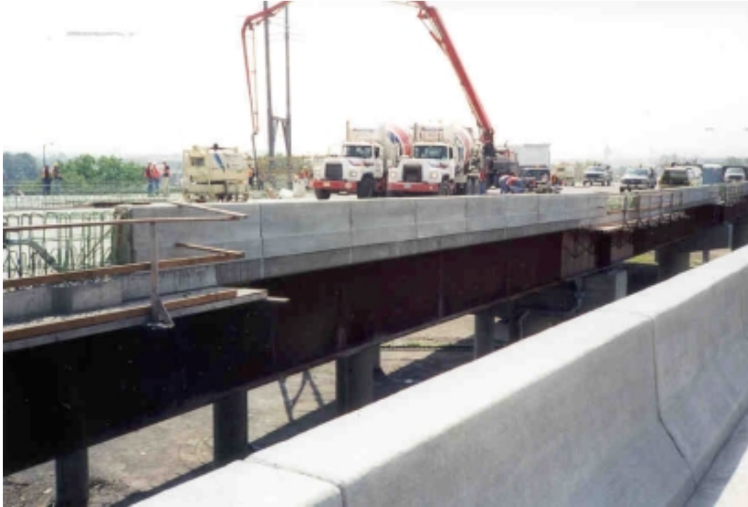
Figure 91. Construction vehicle traffic on the bridge (Bridge No. 0713-151).
