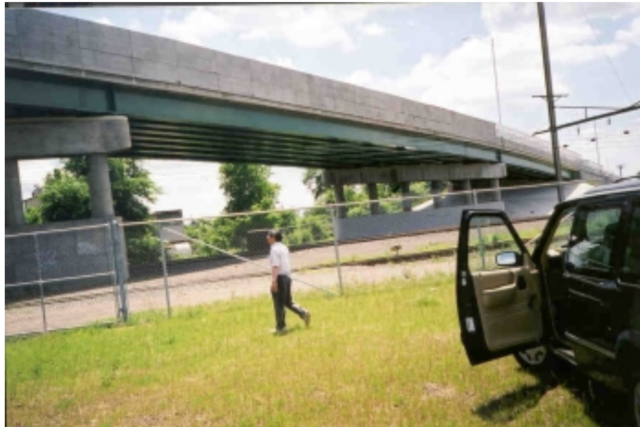
Figure 117. A view of the bridge (Bridge No.1149-168).
