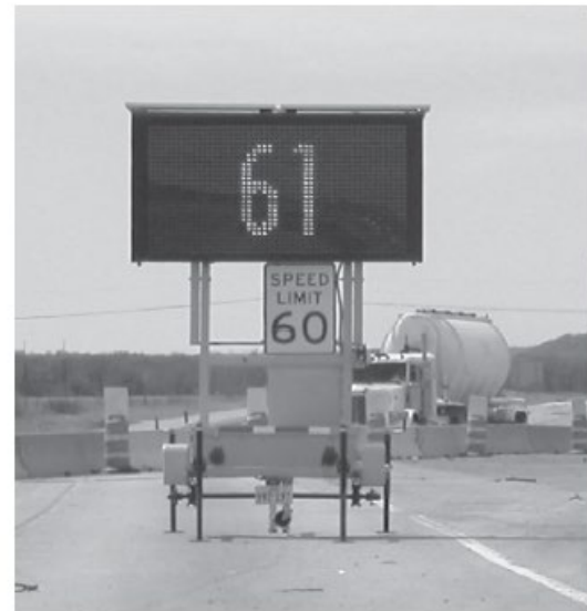
Figure B3. Mobile, lighted, DSFS with multiple messages prior to display of speed – no flashing. [(a) default DSFS message for non-violations; (b) first pass phase for violators; (c) second pass phase for violators; and (d) final phase for violators.] (Brewer et al., 2006)
