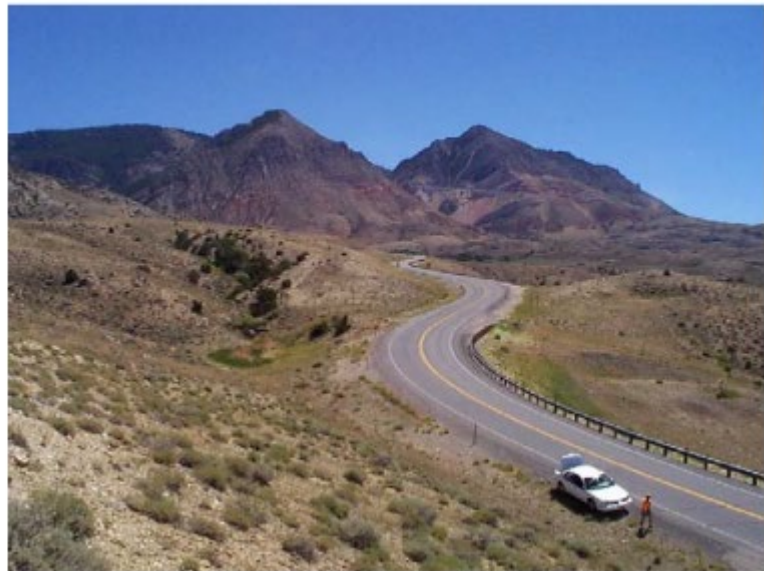
Static Sign (left) and Sharp Curves (right)
