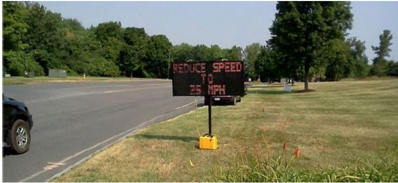
Figure B1. Static, lighted DSFS on CMS that does not display speed and does not flash. (Display activated when speed is greater than 30 mph.) (Bullough et al., 2012)
