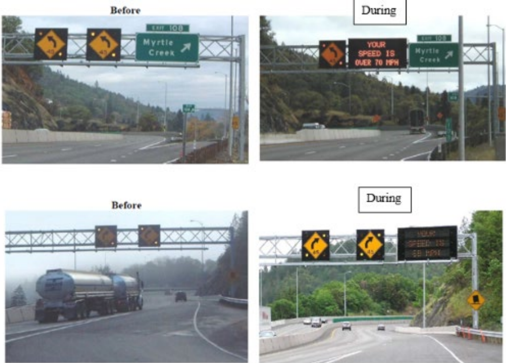
Northbound sign bridge, I-5 Milepost 108.00, before and after ACWS installation
