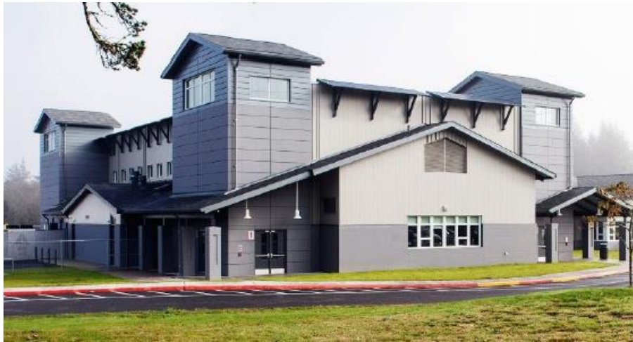
Figure 3.3 Vertical evacuation facility of Westport – Ocosta School gymnasium (25)
