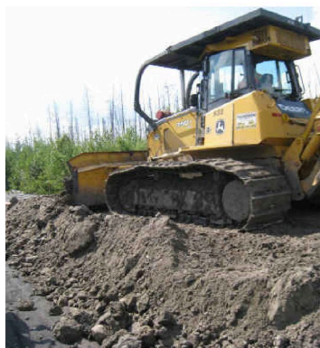
E. Second layer of geocells filled with gravel
