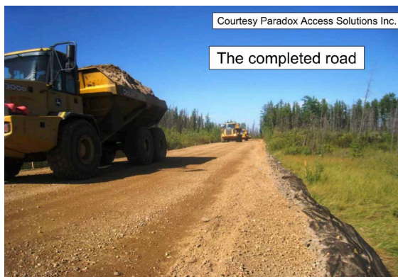
F. Completed road
