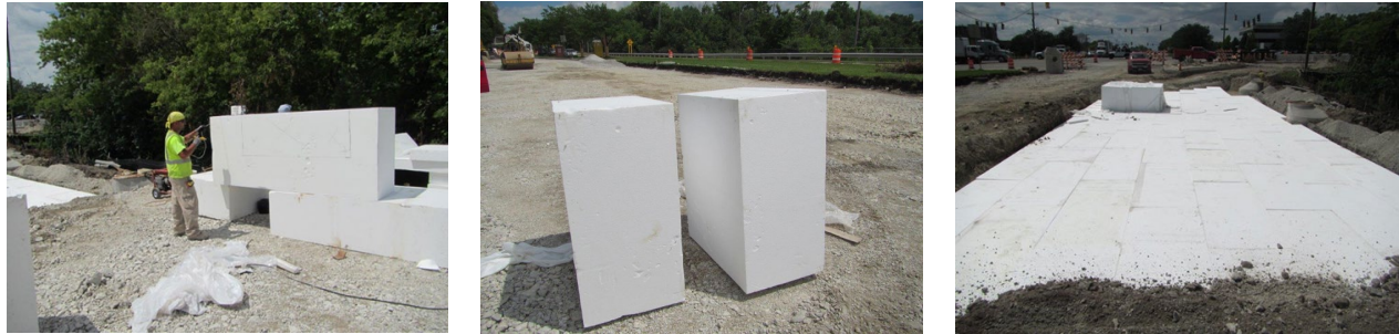
Figure 5. Photos. Using geofoams on IDOT’s contract no. 60W55.
