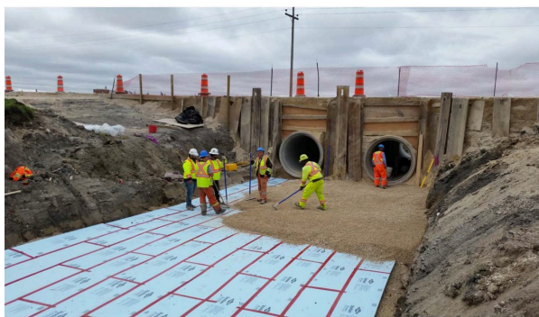
A. Geofom insulation installment
