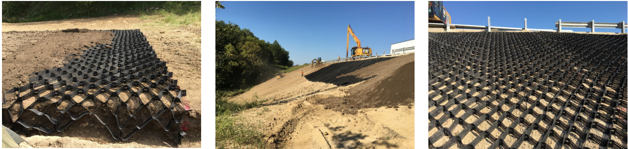
Figure 4. Photos. Soil stabilization using the cellular confinement system (District 7).
