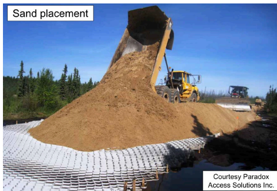
C. Filling with local sand
