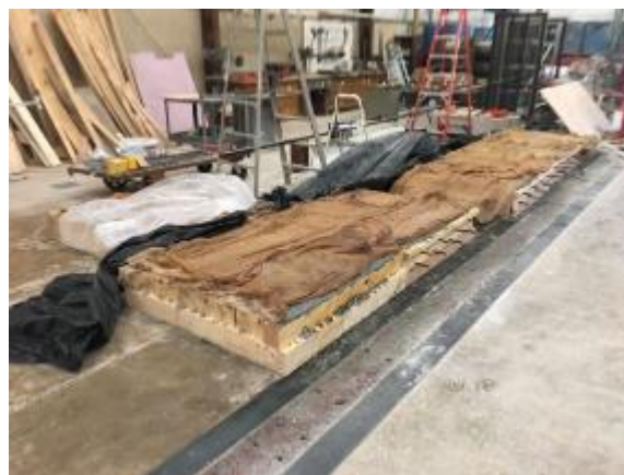
Figure 81. Conventional concrete slabs curing under wet burlap
