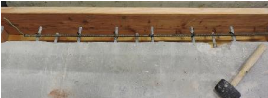
Figure 299. Large-scale corrosion joint specimen with longitudinal connection bar in place
