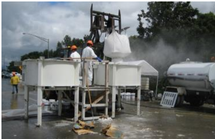
Figure 1. UHPC field mixing operations using high shear mixers (Graybeal 2014)
