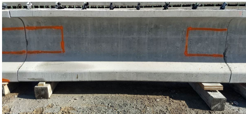
Figure 16. Cut beam segment marked for controlled damage (Shafei, 2020)
