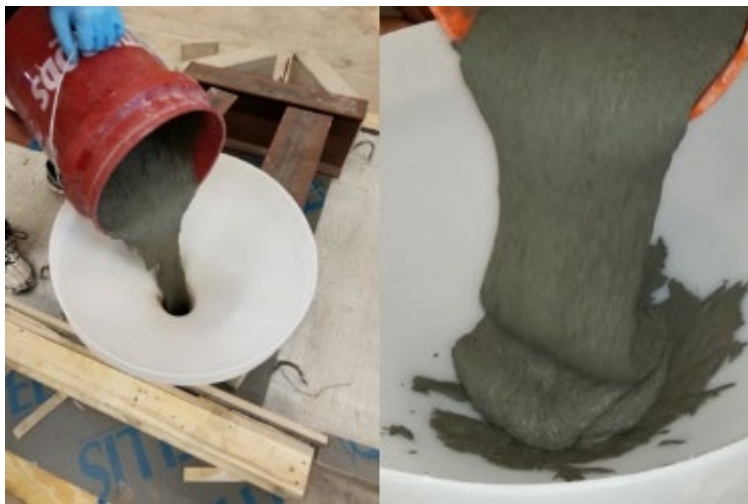
Figure 83. Placement of UHPC into the slab joint formwork
