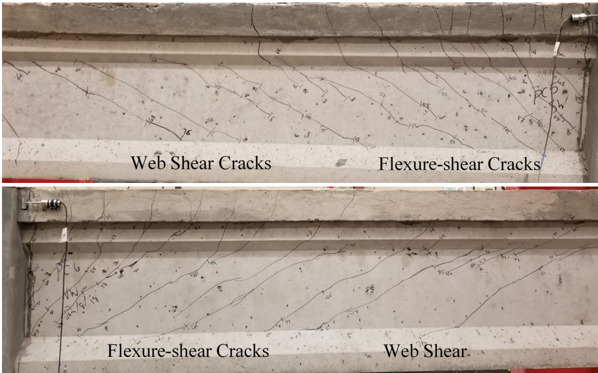
Figure 233. RC1-N girder with flexure-shear cracks and web shear cracks at failure (top) and RC1-S girder with flexure-shear cracks and web shear cracks at failure (bottom)
