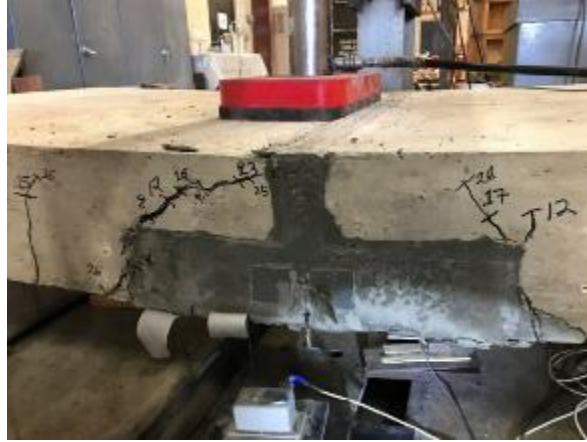
Figure 140. Large cracks at the conventional concrete to UHPC interface after part 1 of testing for Ductal® slab joint 1
