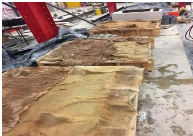
Figure 95. Concrete slabs curing covered by wet burlap
