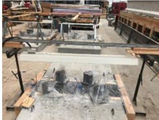
Figure 102. Heat curing of OU J3 half-depth slab joint specimens
