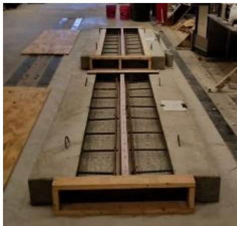
Figure 340. Demonstration joint specimens before UHPC placement
