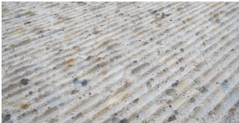
Figure 3. Final bridge deck substrate preparation (Graybeal 2017)
