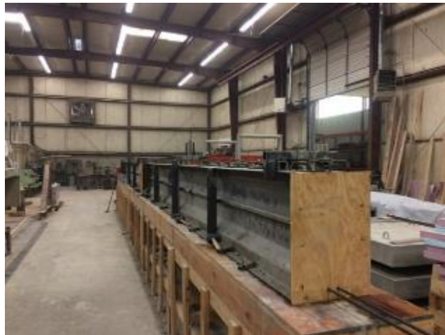
Figure 173. Prestressed beam formwork immediately before casting
