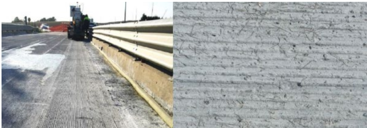
Figure 6. Finished overlay on the Mud Creek bridge (Wibowo and Sritharan 2018)
