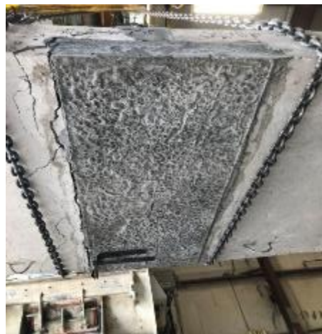
Figure 153. Cracks on the as-tested underside of Ductal® slab joint 2 after testing
