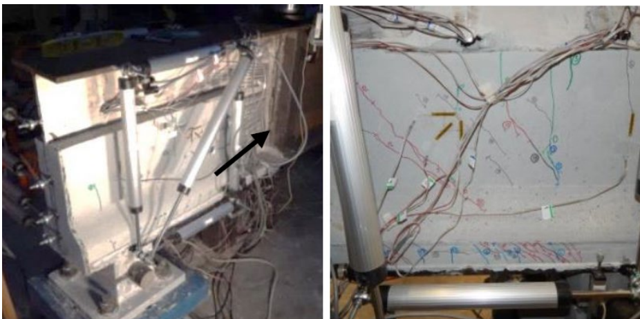
Figure 15. Repaired girder failure (Zmetra 2015)
