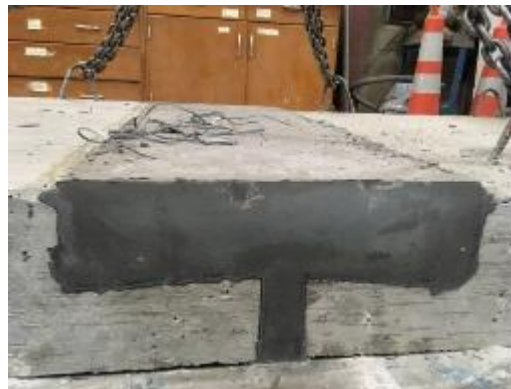
Figure 103. Completed half-depth slab joint cast using OU J3 mix
