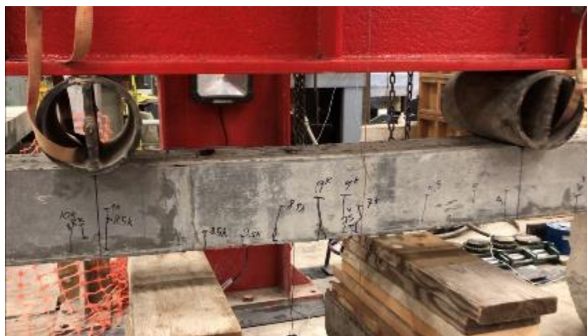
Figure 76. Crack pattern for test SB-D5-2
