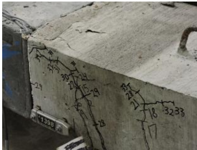
Figure 117. Slab joint at failure showing concrete crushing on the compression face, cracking in base concrete, and opening at joint interface
