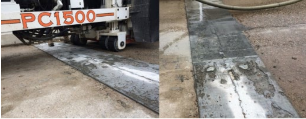
Figure 332. UHPC joint before (left) and after (right) grinding
