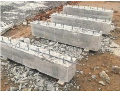
Figure 298. Large-scale corrosion joint specimens after chipping
