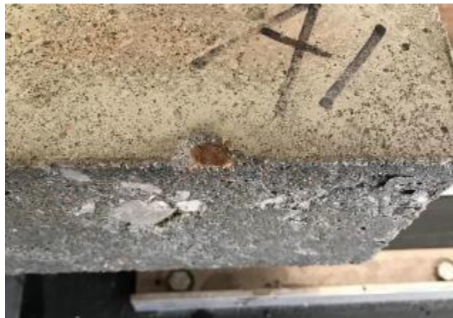
Figure 277. Deteriorated state of a class AA freeze-thaw specimen - Cycle 350
