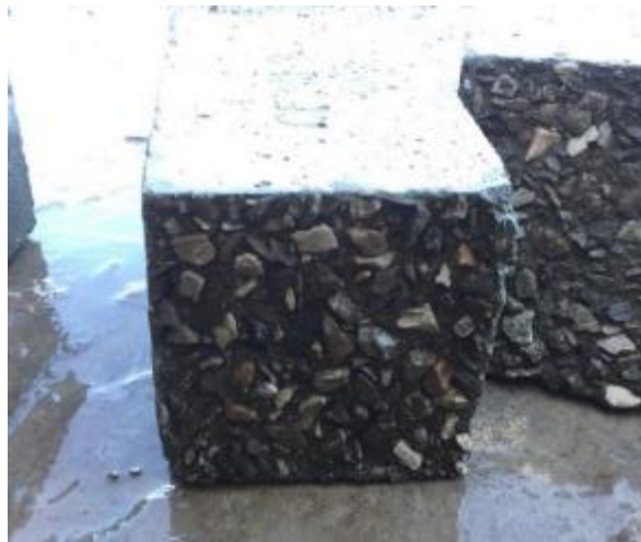
Figure 53. Exposed aggregate surface after power washing
