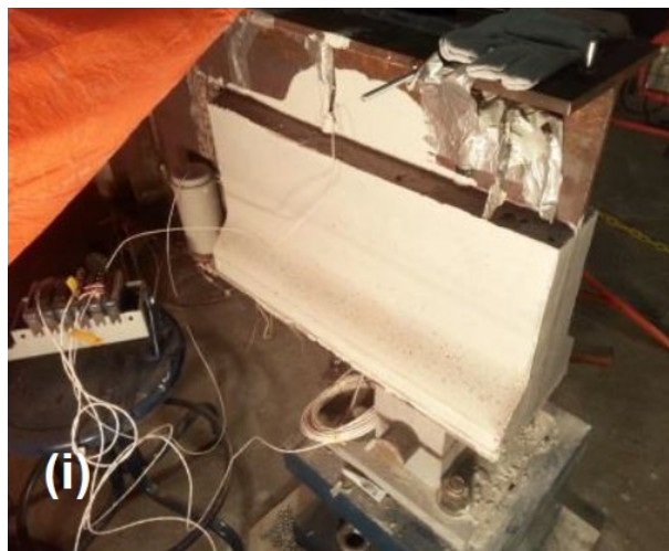
Figure 12. Final repaired girder (Zmetra 2015)
