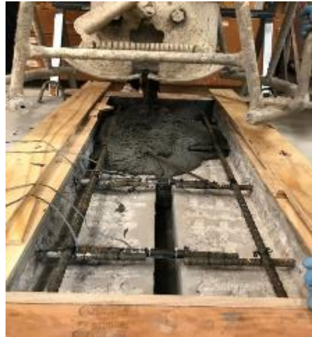
Figure 100. Placement of UHPC connecting two slab panels
