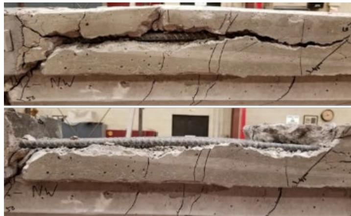
Figure 214. NC2-S girder before excavation of the concrete in the deck (top) and the deck after excavation exposing the reinforcement (bottom)
