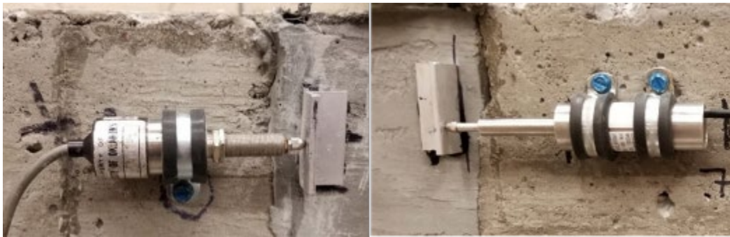
Figure 192. LVDTs used to measure joint separation attached to the girder
