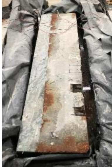
Figure 305. Joint corrosion in Ductal® large-scale corrosion specimen during week 5 of testing
