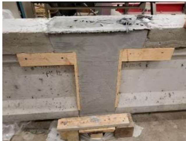
Figure 188. Completed continuity joint representing new construction
