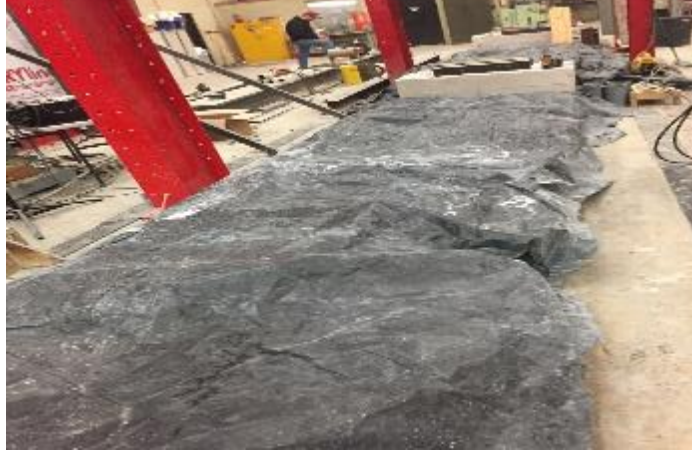
Figure 96. Plastic tarp covering curing concrete slabs
