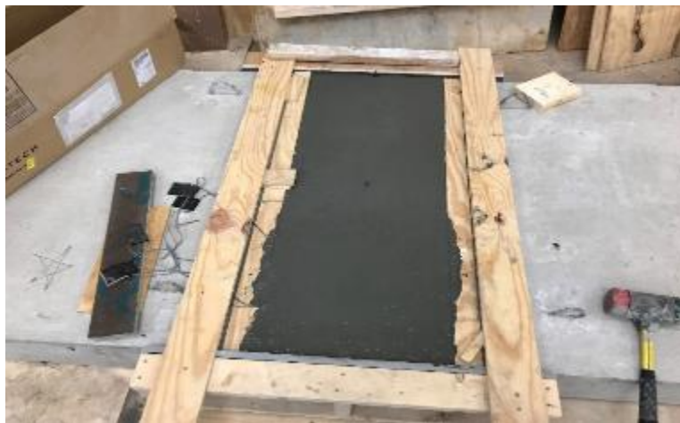
Figure 101. Self-consolidating UHPC filling the joints
