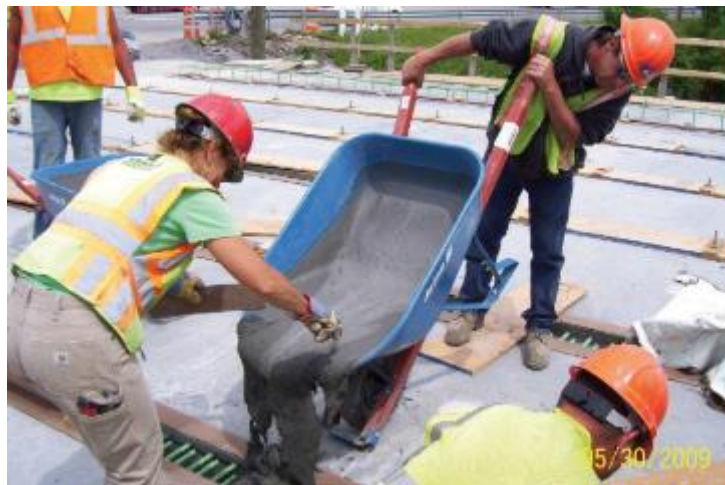
Figure 2. UHPC placement into a longitudinal connection of bridge elements (Graybeal 2014)
