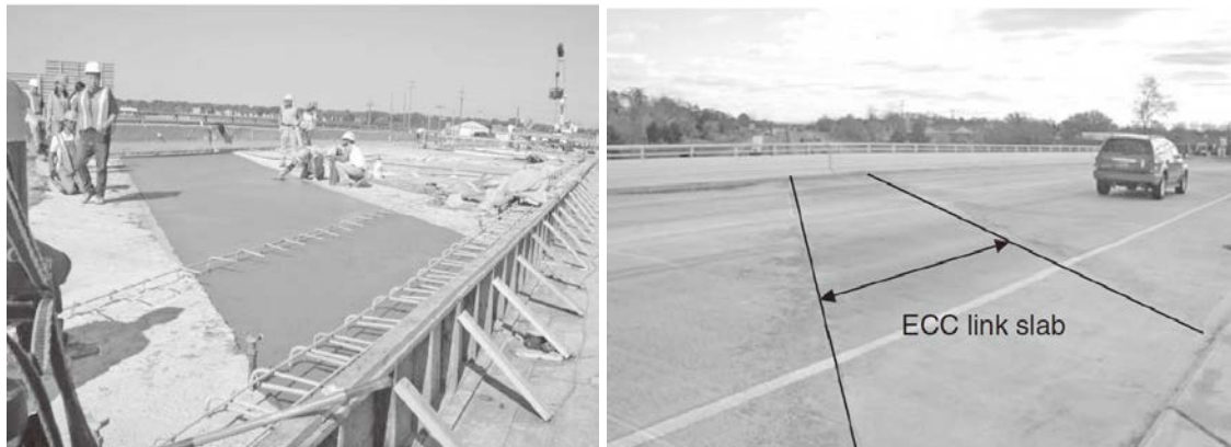
Figure 5-4 ECC Link Slab Constructed in Michigan (Li 2014)
