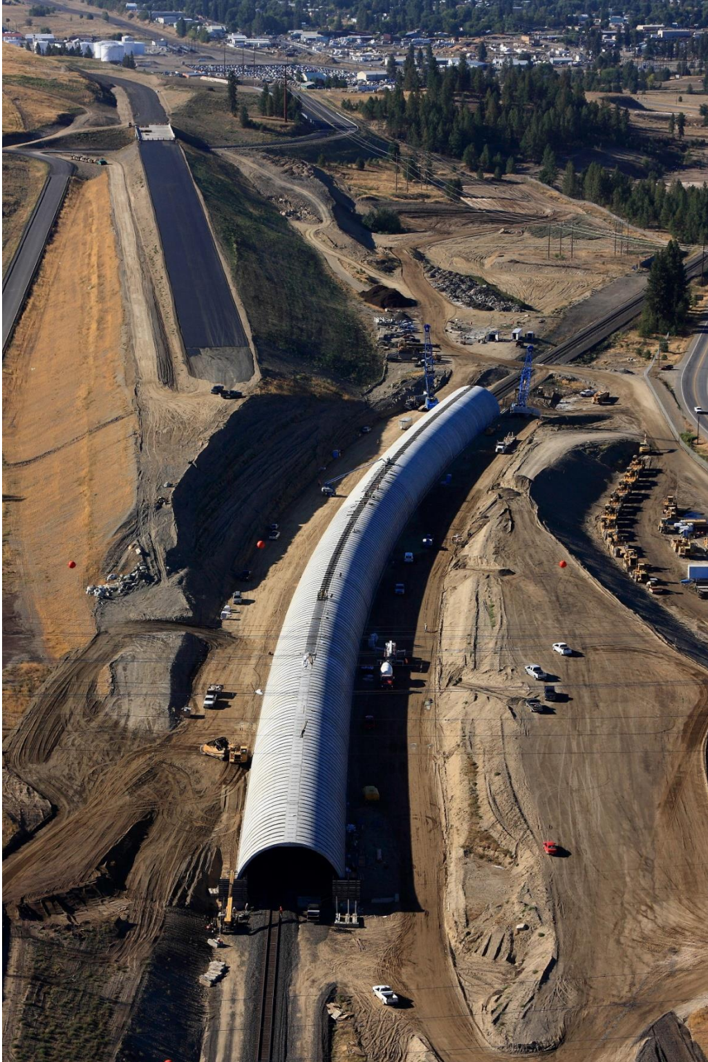
Figure 10. Overview showing arch and fill under construction.
