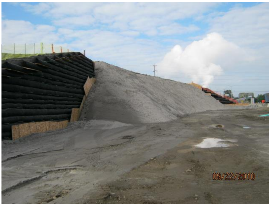
Figure 17. P-line Bridge Pre-load between Abutments (Sites No.10 and No.11).
