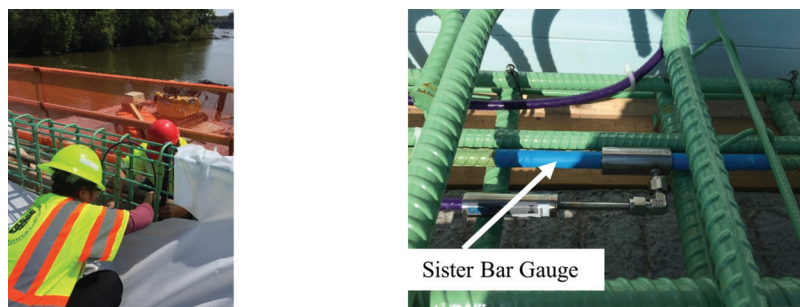
Figure 3.3 Researchers installing a sister bar gauge in Asset 331-71-08732 (left) and the installed gauge (right).
