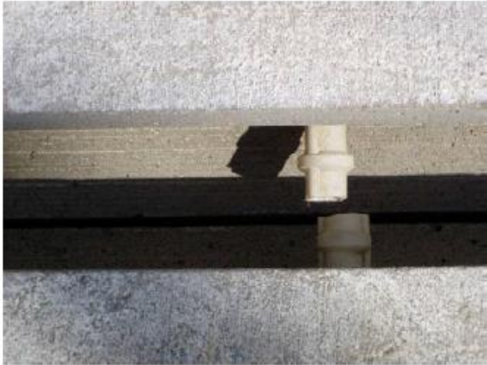
Misalignment of ducts
