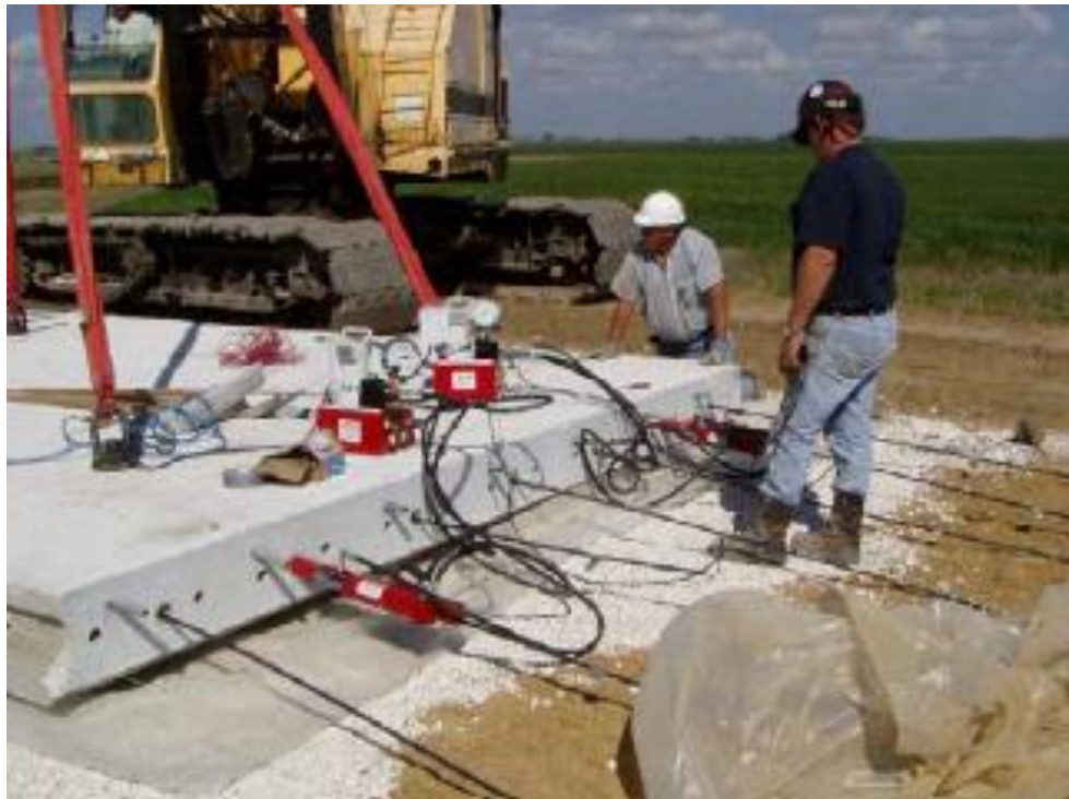
Stressing longitudinal post-tensioning strands
