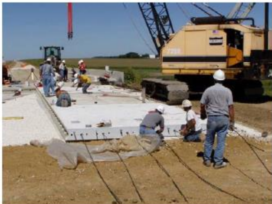
Threading longitudinal post-tensioning strands
