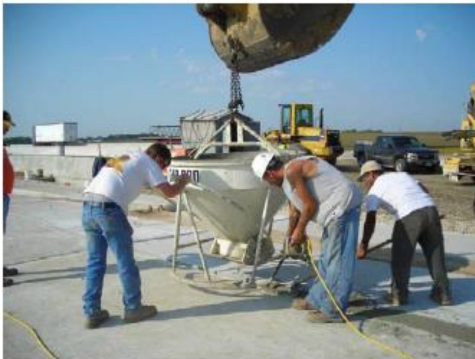
Casting longitudinal joint
