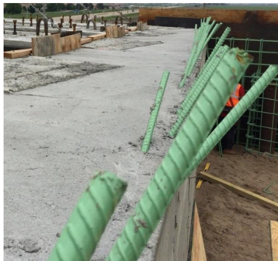
Figure 4.23: Current practice of using #6 @12 in. dowels to connect approach slab at the abutment
