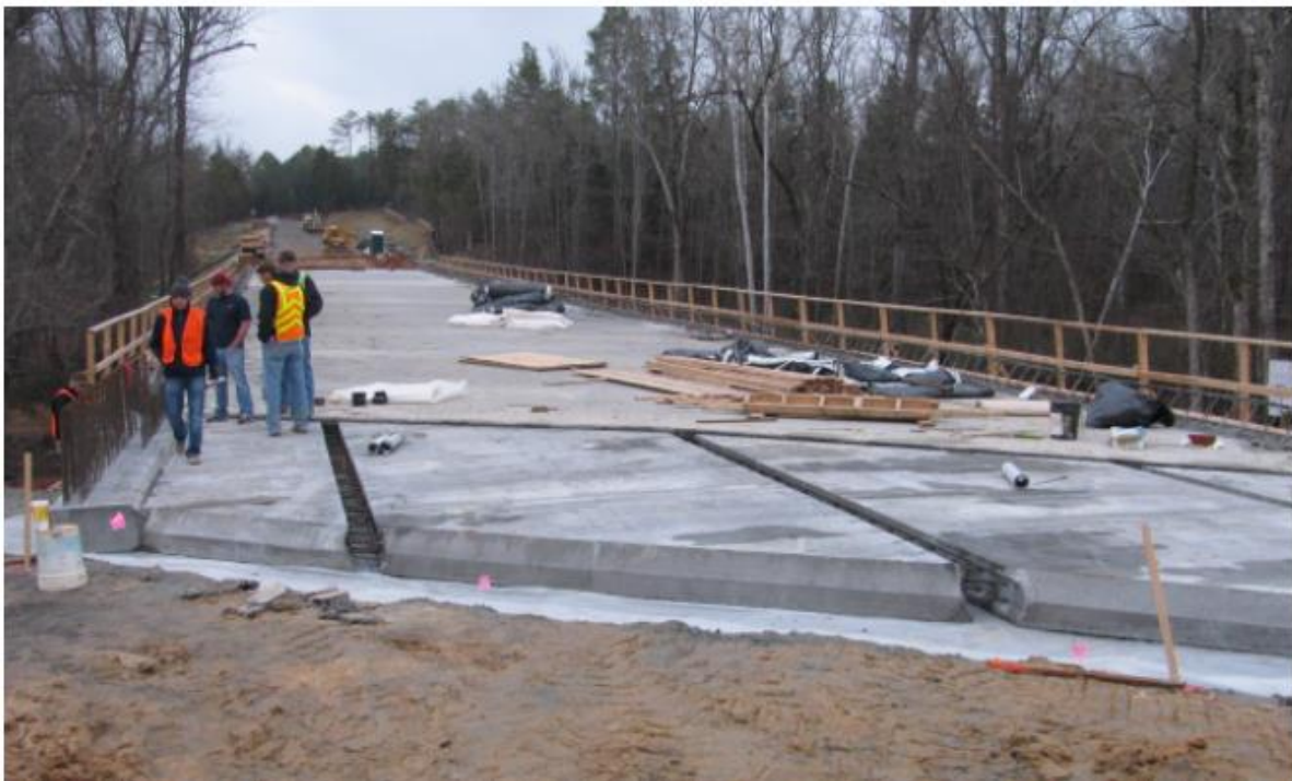
Complete installation of skewed panels
