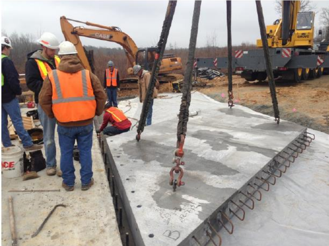
Panel installation over polyethylene sheeting
