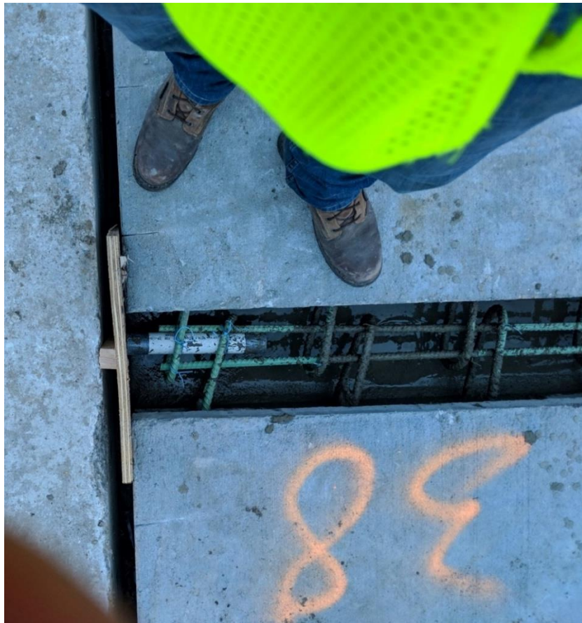
Precast panel joints and connections
