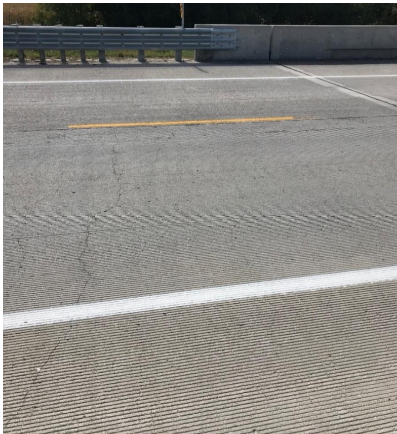
Figure 3.5: Cracking map of approach slab and paving section of Little Sandy Creek bridge.
