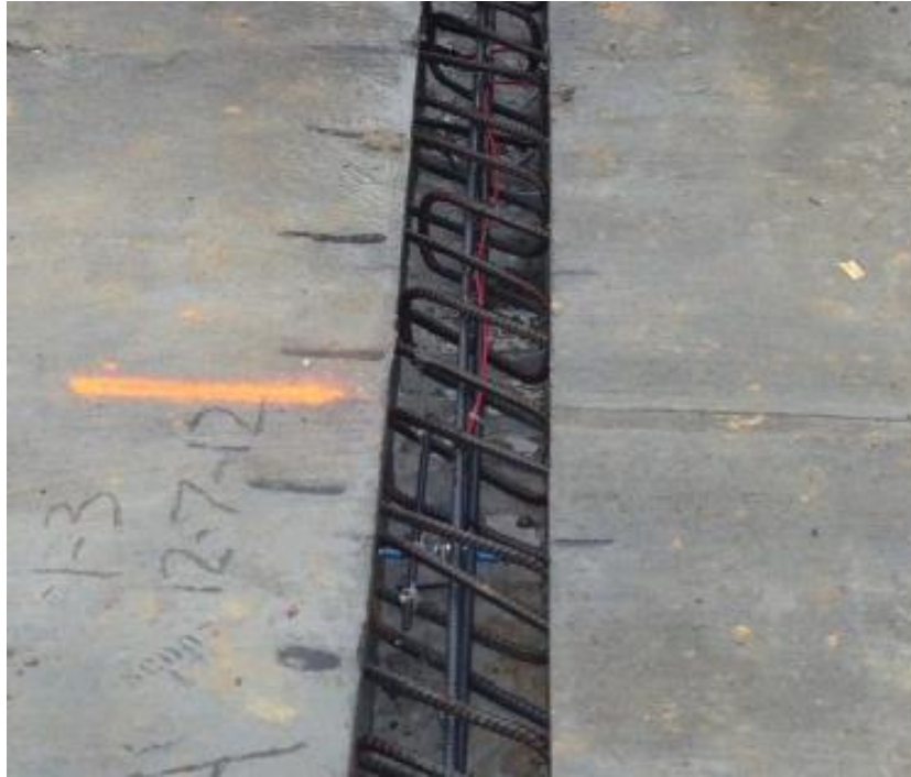
Reinforcement of longitudinal joints
