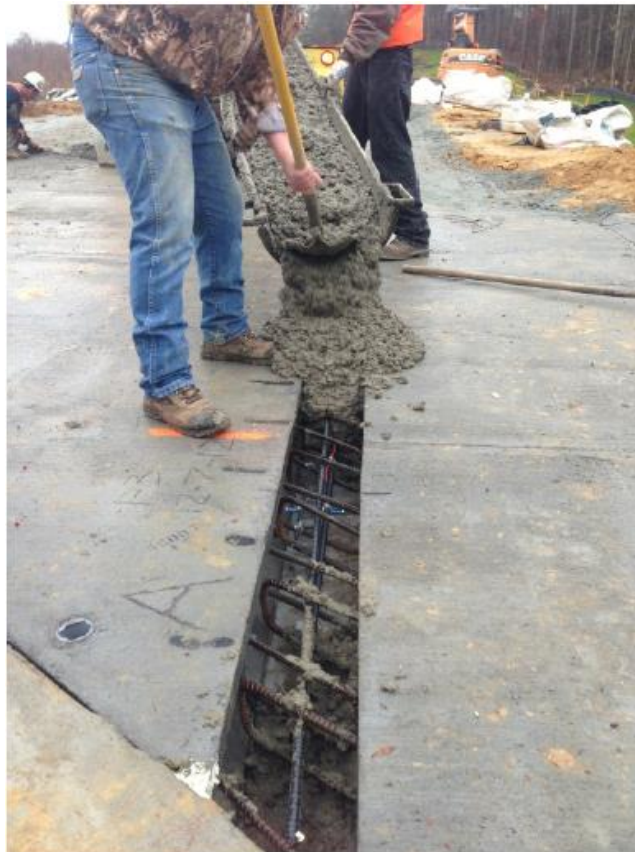
Casting longitudinal joints
