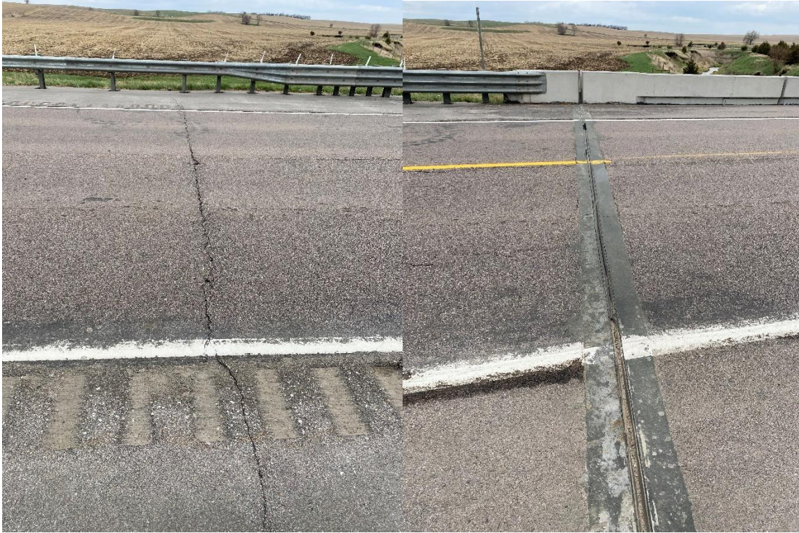
Asphalt cracking at the end of paving section (left) and expansion joint (right)
