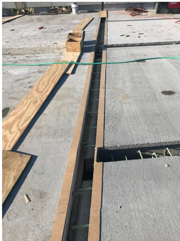
End of Floor Connection
