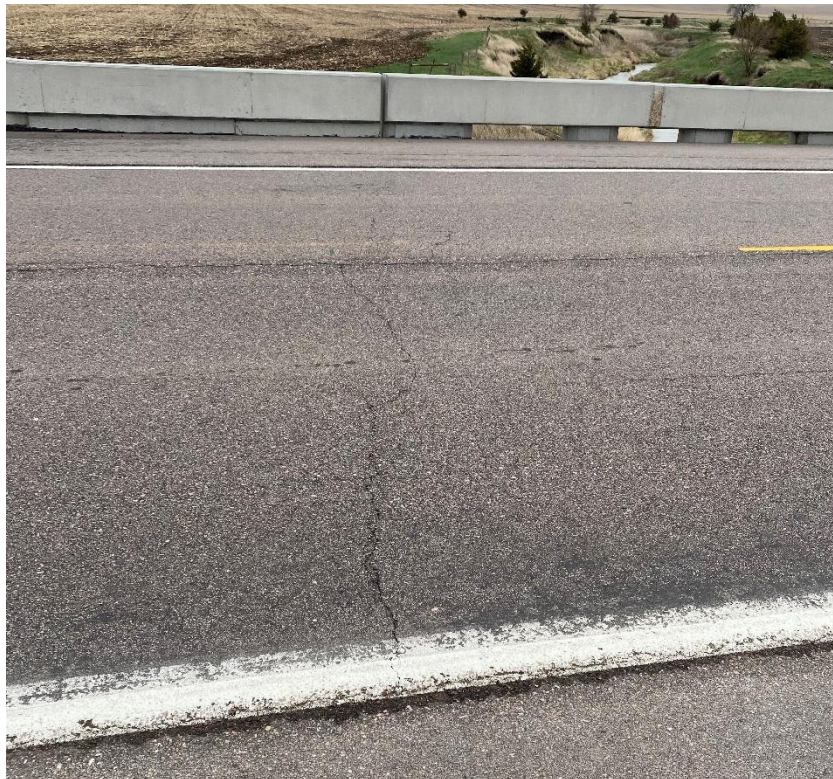
Asphalt cracking at the end of floor
