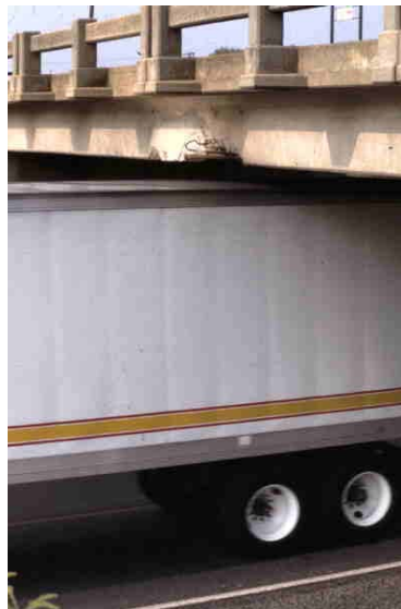
Figure 4.6. Vertical clearance for vehicles at grade separations.
