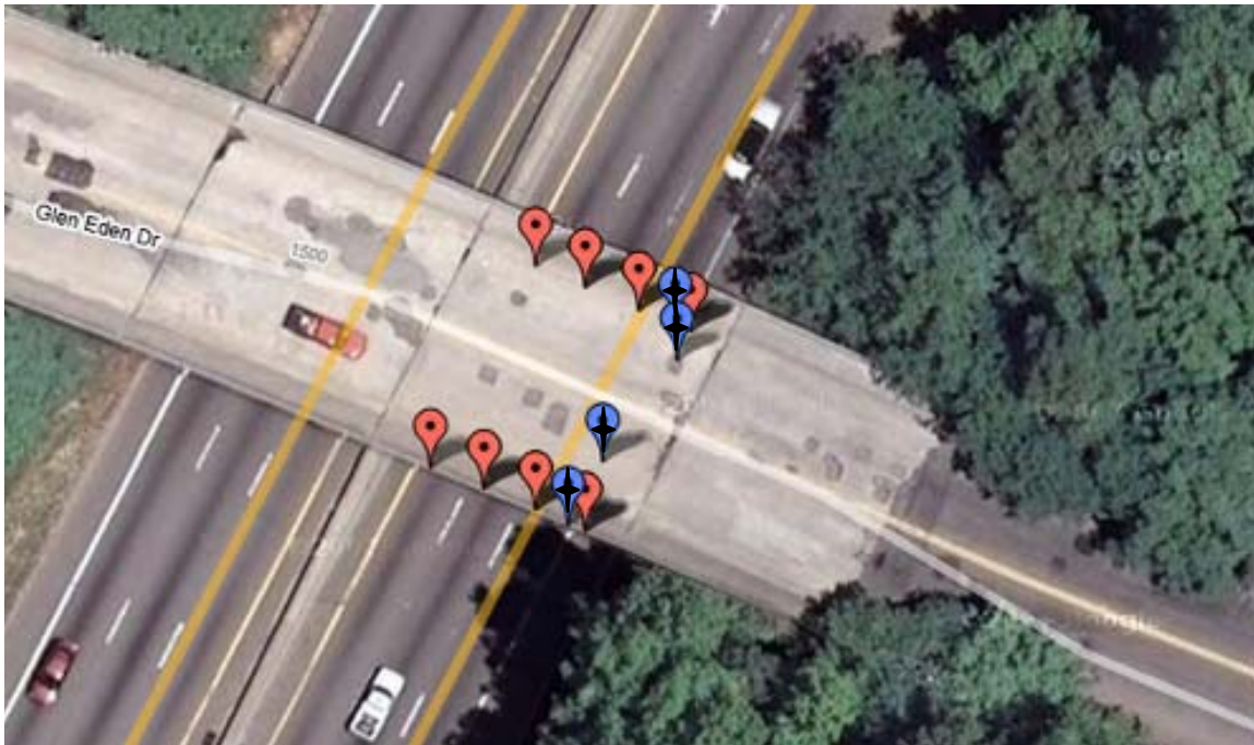
Figure 4.13. Survey and Geo-3D measurement locations for Glen Eden Drive bridge.
