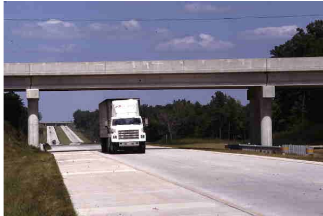
Figure 4.5. Bridge vertical clearance at grade separations.
