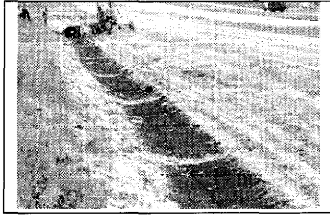
Figure 31. Installed synthetic mat channel lining.
