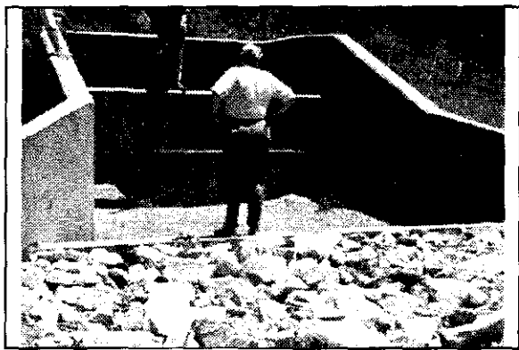
Figure 51b. Baffle-wall energy dissipator - USBR Type VI.
