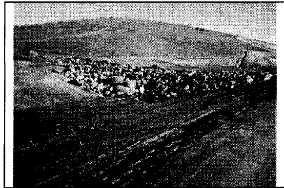
1.8t Rock-riprap drop structure
