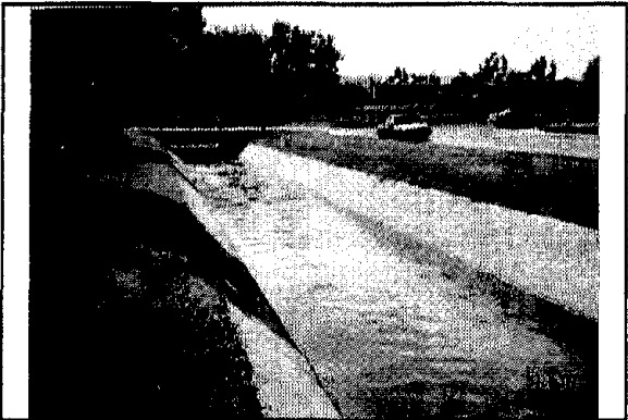
1.8c Concrete-lined channel
