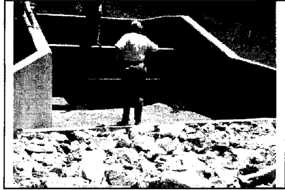
1.8r U.S. Bureau of Reclamation (USBR) impact basin energy dissipator
