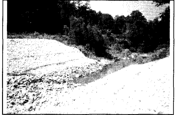
5.10b Riprap channel lining
