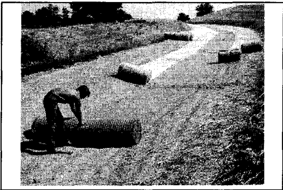
5.10c Straw blanket temporary lining
