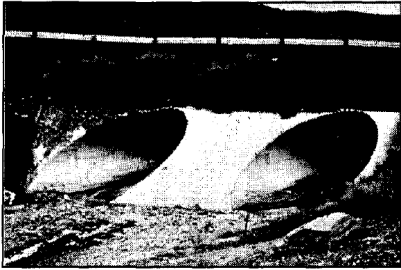
7.5a CMP culvert
