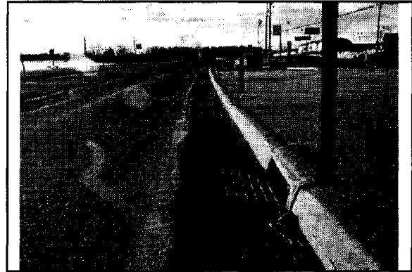
7.56 Inlet before turn lane
