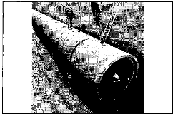
7.4b Installing storm drain pipe
