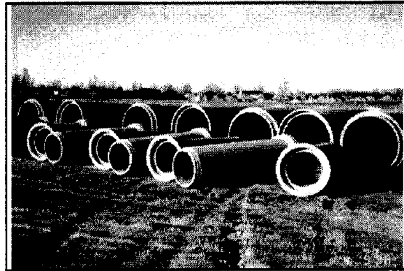
1.8l Storm drain pipe
