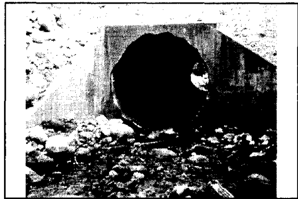
7.14 Cast-in-place headwall
