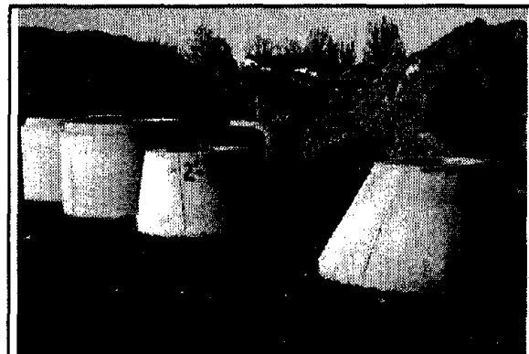
6.15 Precast concrete access hole components prior to installation
