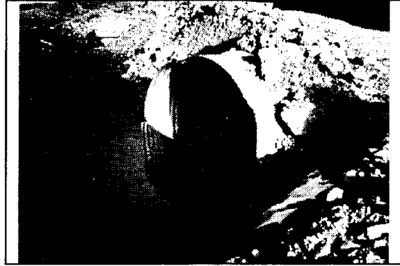
8.7 Flow conditions at culvert inlet
