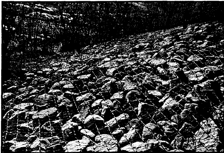
Figure 3.2 Wire enclosed riprap used for guide bank side slope protection at I-25 crossing of Rio Galisteo, New Mexico (NMSHTD)
