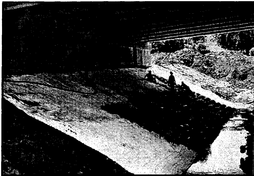
Figure 5.3 Installation of articulating block mat proceeding upslope (ODOT)
