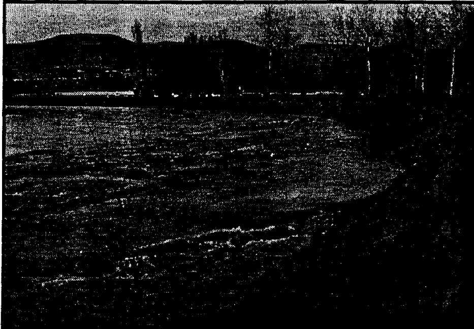
Figure 1.7 Submerged bendway weirs on the Yakima River, Washington at high flow (WSDOT)
