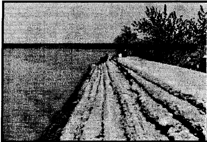
Figure 2.1 Stair step facing on Bonny Reservoir, Colorado after 30 years (PCA).
