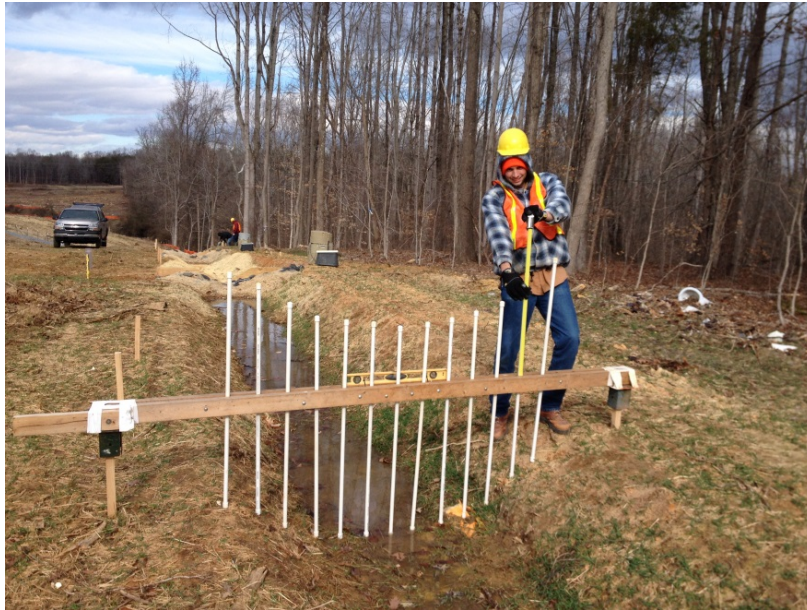
Figure 7. Using the cross-section pin measurement device in a bare soil (control) treatment section of the ditch.
