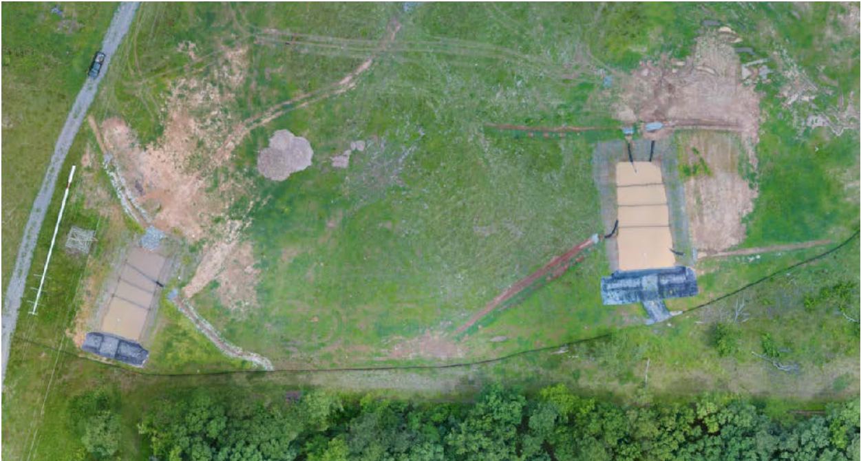
Figure 17. Posi-Shell-lined basin on left and unlined inlet basin on right illustrating potential effects on turbidity.
