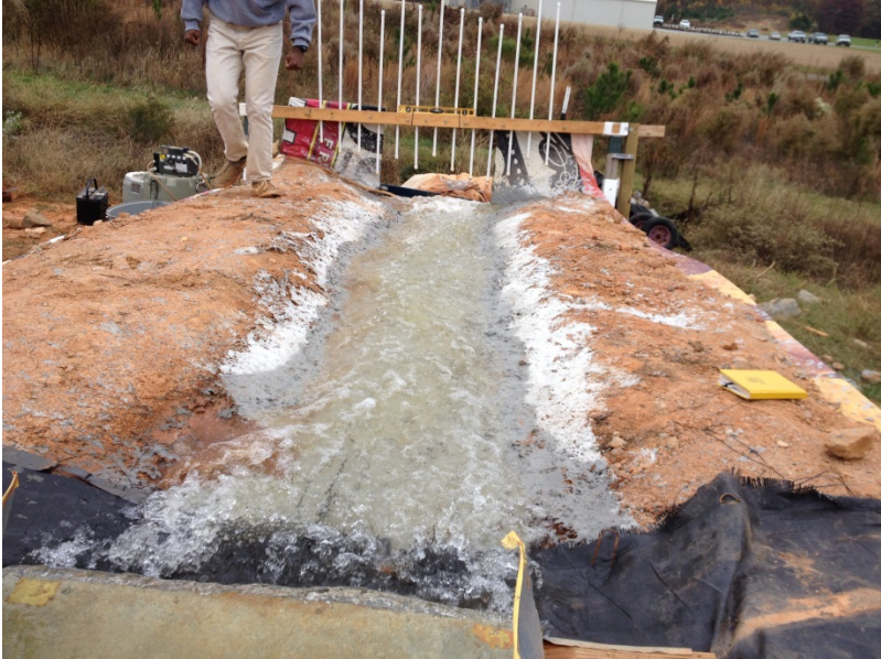
Figure 5. Testing the hydraulically applied concrete product with a 1 cfs test flow.
