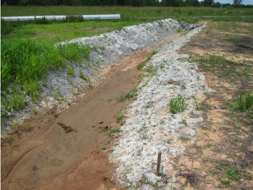
Figure 13. Posi-Shell-lined ditch in May 2017, one month after application.
