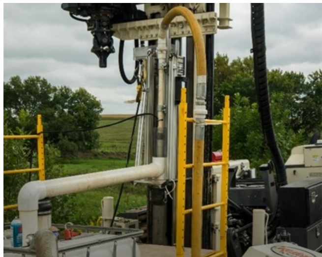
The ISTD equipment assembled in front of the drill rig.
