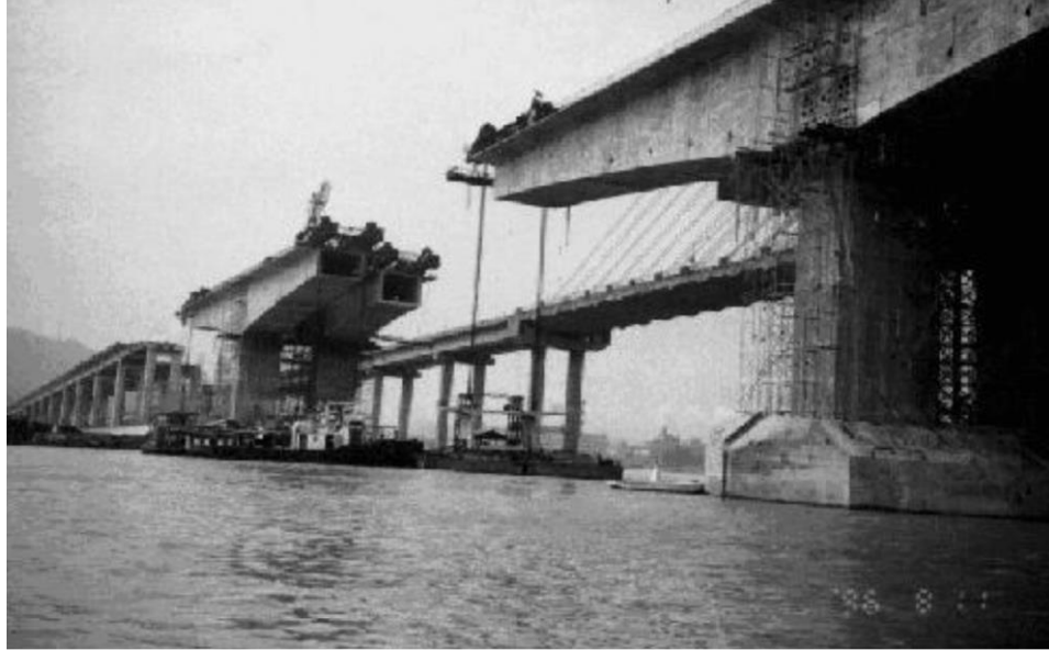
Figure 2.51. Second Jiujiang Bridge (Li et al. 2008)
