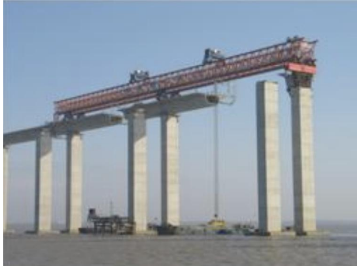
Figure 2.53. Launching gantry adopted for construction (Li et al. 2008)
