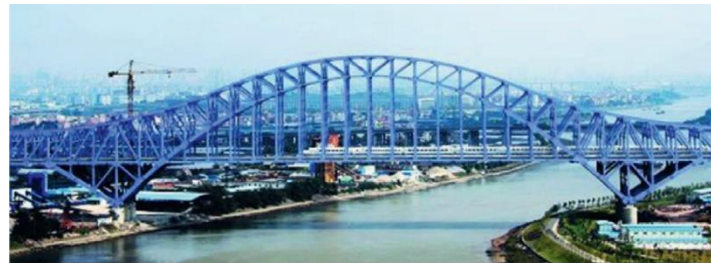
(a) Dongping Bridge
