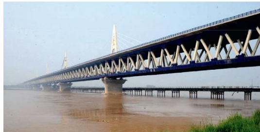
(c) Zhengzhou Bridge
