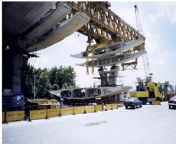
Figure 2.49. Humin Viaduct construction (Li et al. 2008)
