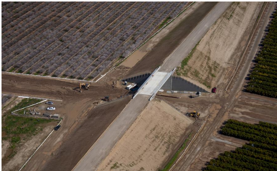
Figure 2.62. A construction site from Merced to Bakersfield route (ENR 2019)
