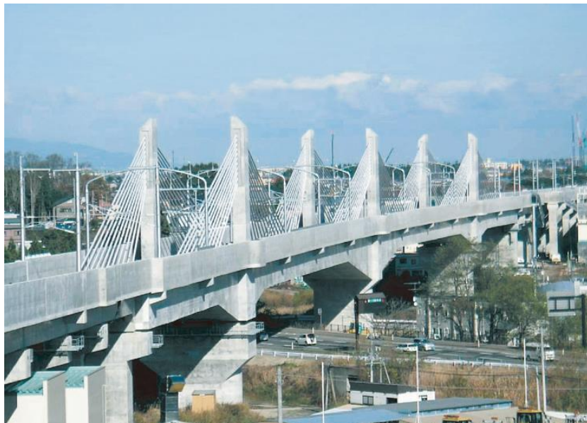
Figure 2.2. Sannai Maruyama Bridge in Aomori, Japan (Zenitaka 2010)
