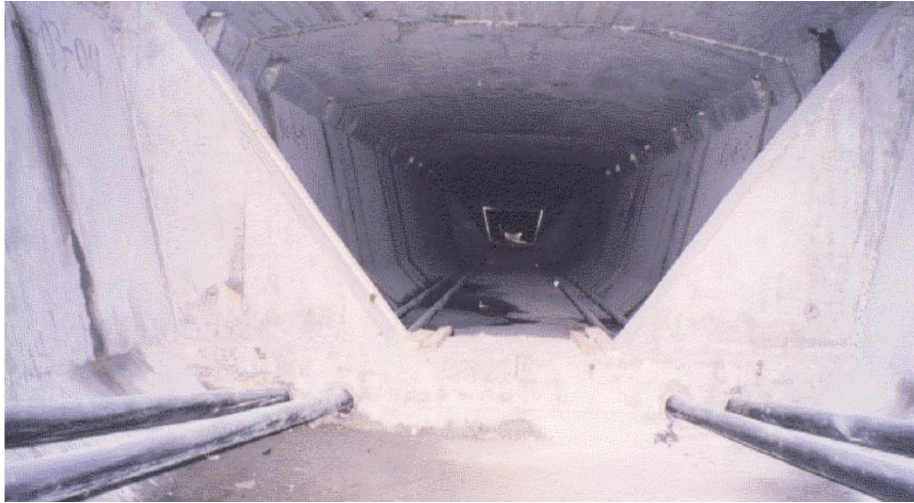
Figure 2.48. Installed tendons in Liuhe river bridge (Li et al. 2008)
