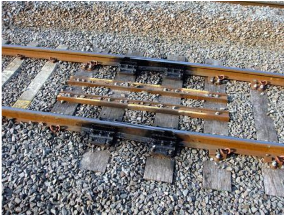
Figure 2.30. Rail expansion device (Connor 2019)
