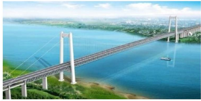
(b) Wufengshan bridge
