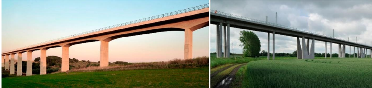
Figure 2.22. Integral HSR bridges (Su et al. 2019)
