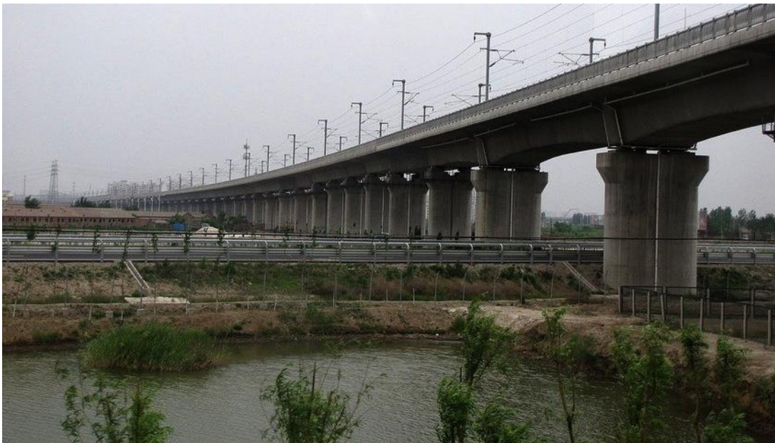
Figure 2.19. Beijing-Tianjin HSR bridge (Sweet 2014)
