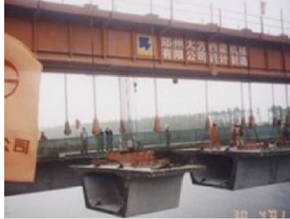
Figure 2.47. Liuhe river bridge (Li et al. 2008)
