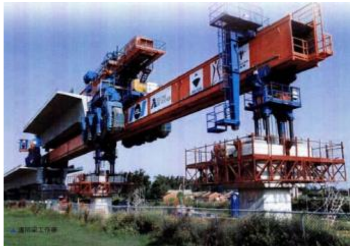
Figure 3.11. Transporter with hoisting equipment used in Taiwan (Tai et al. 2010)
