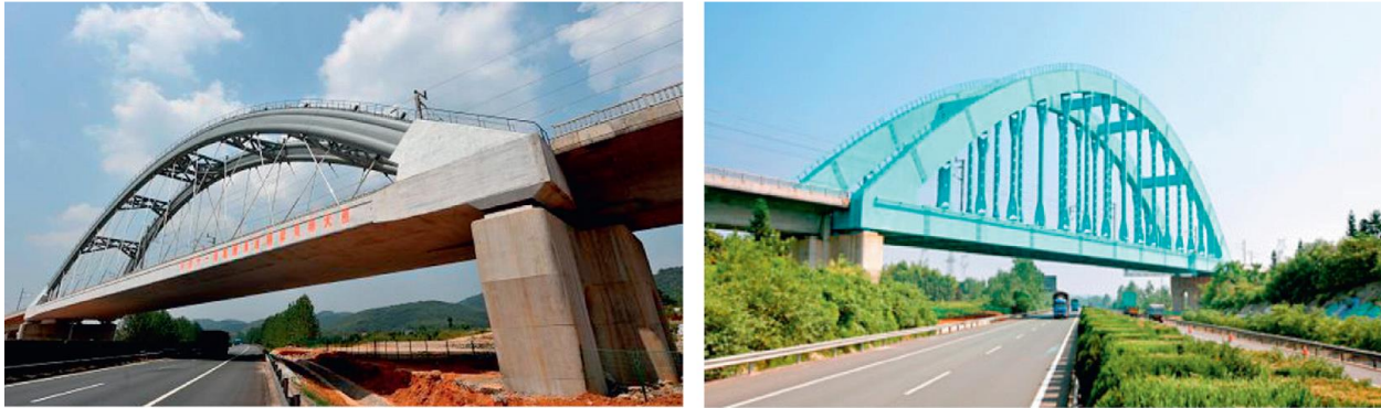
Figure 2.41. Tied steel arch HSR bridges: (a) Hujawan Bridge and (b) Tingsihe Bridge (Hu et al. 2014)
