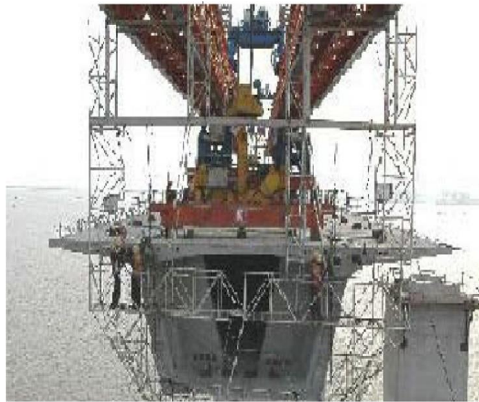
Figure 2.54. Deviator segments placement (Li et al. 2008)
