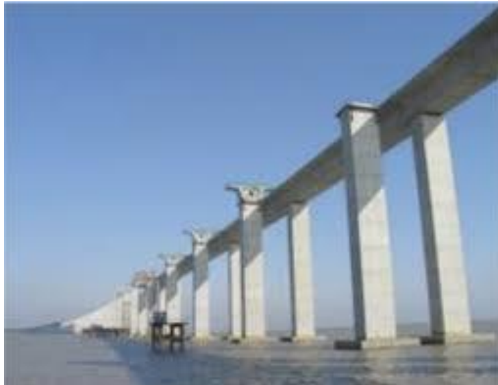
Figure 2.52. Sutong Bridge in deep water (Li et al. 2008)
