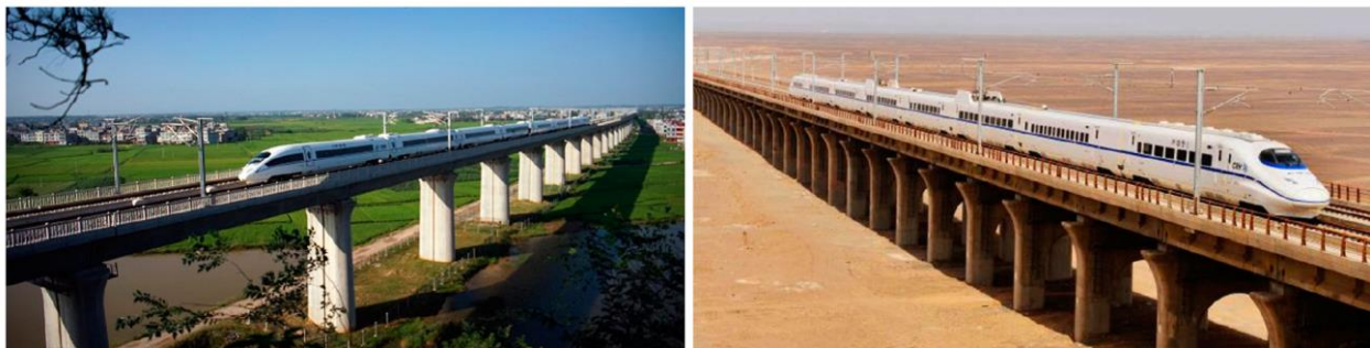
Figure 2.20. Examples of simply-supported bridges in China (Su et al. 2019)
