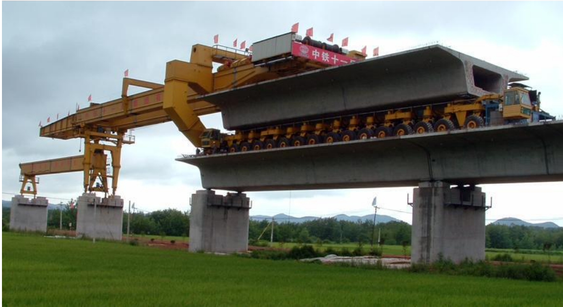
Figure 2.50. Full span pre-casting (Rosignoli 2016)
