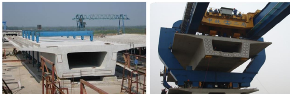
Figure 2.33. Precast and erection (Yan et al. 2015)
