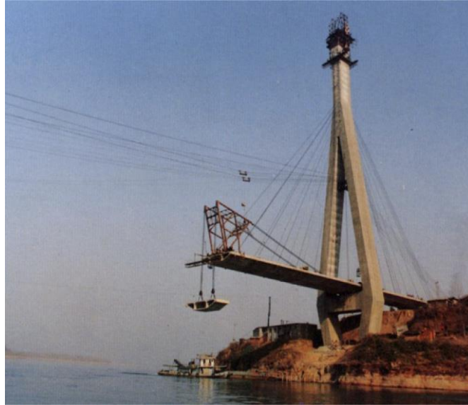
Figure 2.55. Yunyang Bridge under construction (Li et al. 2008)
