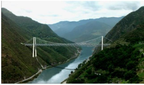
(a) Jinshajiang suspension bridge
