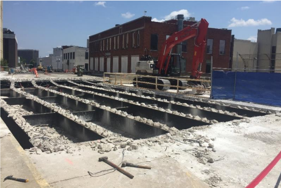
Figure 20. Staged deconstruction of the existing bridge in downtown Atlanta
