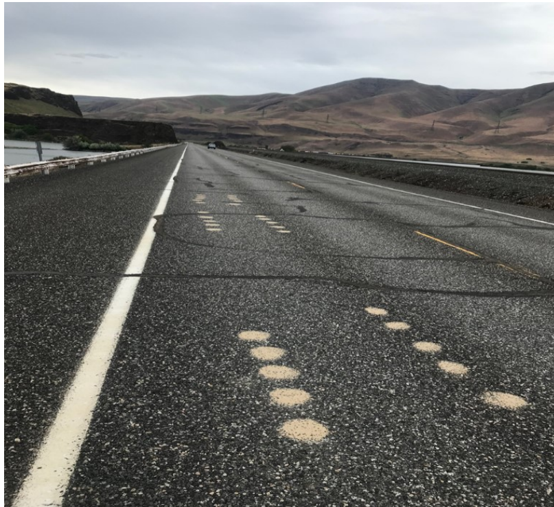
Figure 9.6. Sand circle tests prior to construction
