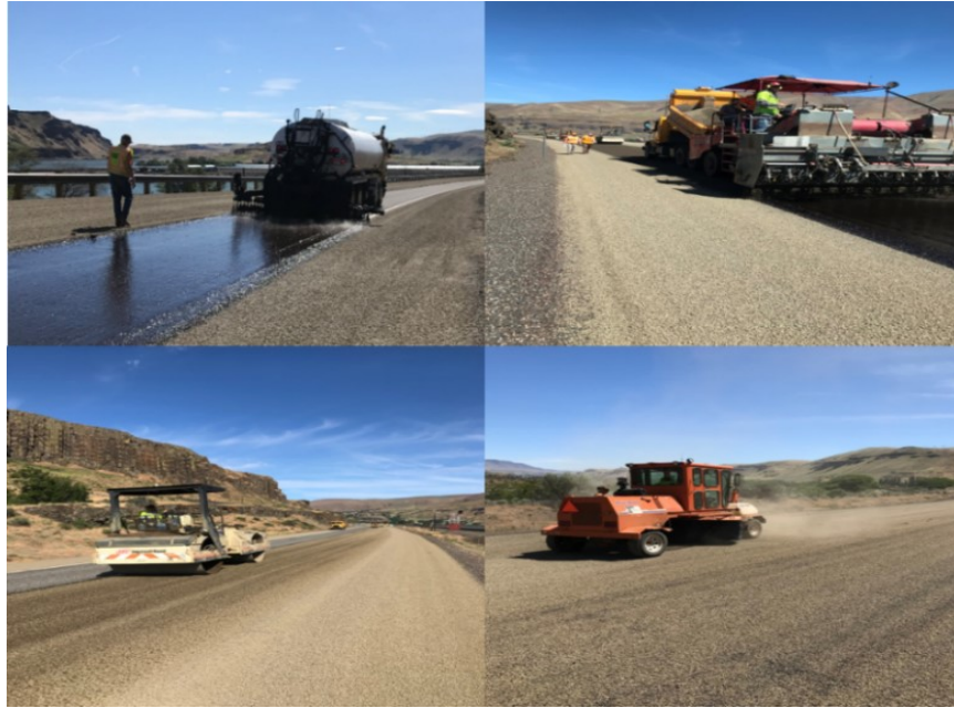
Figure 9.3. Chip seal construction equipment
