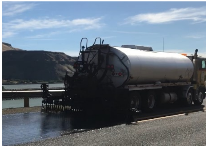
Figure 9.5. Asphalt emulsion spraying for triple coverage
