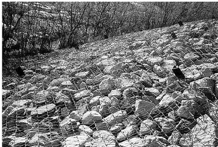
Figure 3.2. Wire enclosed riprap used for guide bank side slope protection at I-25 crossing of Rio Galisteo, New Mexico (NMSHTD).
