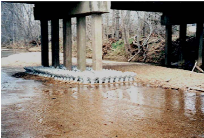
Figure 6.13b. Newly-installed A-Jacks armor units at Bridge 133, Graves County, KY
