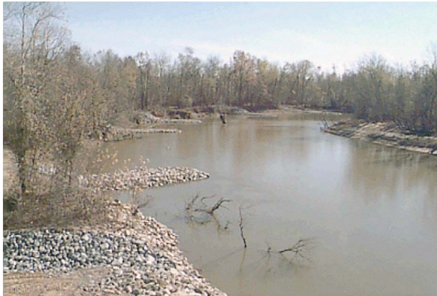
Figure 1.9. Bendway weirs on northbank of Hatchie River looking upstream (TDOT).
