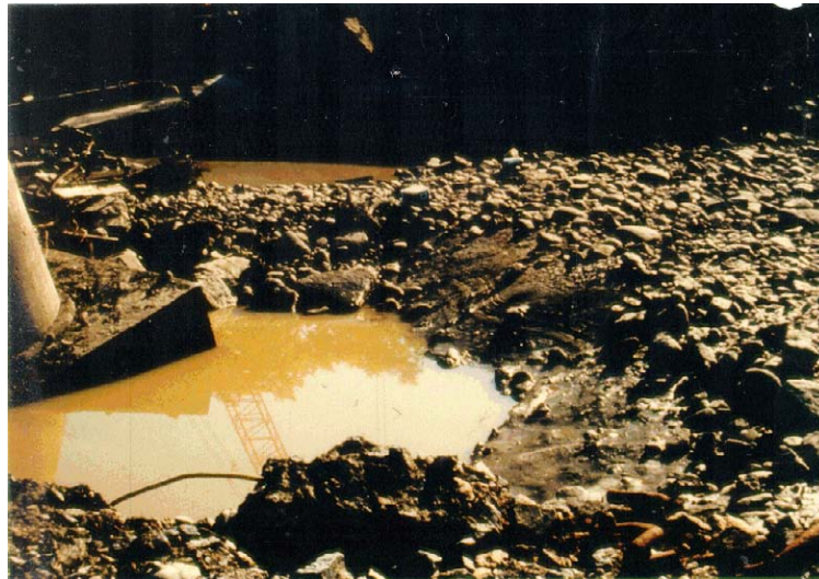
Figure 8.2. Pier scour holes at Schoharie Creek bridge in 1987. Pier 2 in the foreground with pier 3 in the background. (2)
