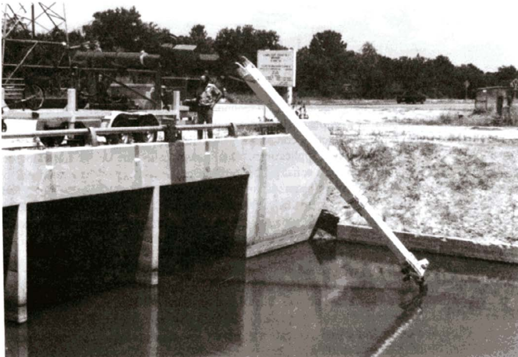
Figure 7.8. FHWA articulated arm in use.
