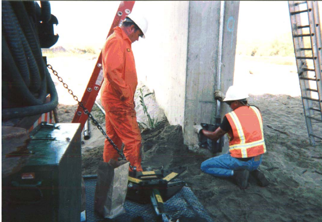
Figure 7.13. Installation of a sonar scour monitor on Salinas River bridge near Soledad, California (Highway 101) by CALTRANS.
