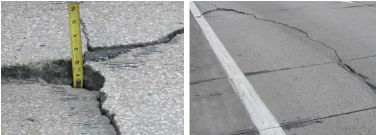
Figure 2.20 An example of problems encountered in the approach slabs in Kansas (Thiagarajan and Gopalarathnam, 2010).
