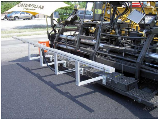
(a) Infrared System Installed on Paver
