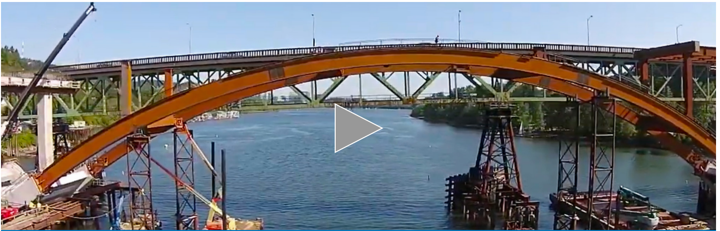
The Sellwood Bridge project in Multnomah County, OR, used CM/GC contracting to incorporate innovations such as slide-in bridge construction and 3D modeling . Watch the old Sellwood Bridge be replaced in this time-lapse video .
